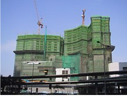
Bamboo scaffolding can reach great heights.
