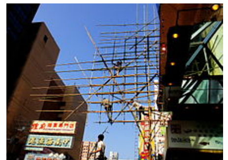
Bamboo has long been used as an assembly material in Hong Kong because of its versatility
