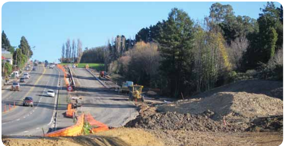
Figure 2. Road widening and realignment work at Caversham. Photo: M. Wakelin.
