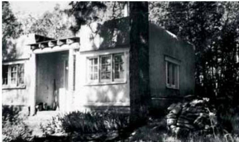
Figure 81. Anchor Ranch, bunkhouse #1, 1943. (Los Alamos National Laboratory)
