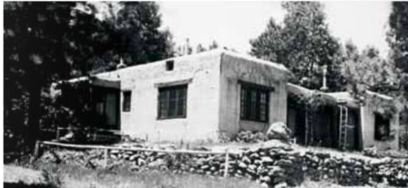
Figure 78. Anchor Ranch main house, 1943. (Los Alamos National Laboratory)
