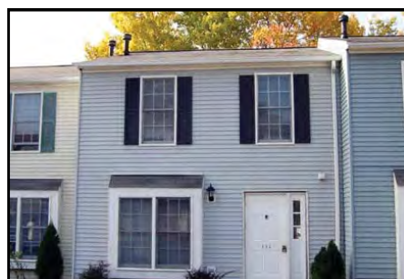
131 Sun Valley $134,900 Remodeled 3BR townhome. All new floor coverings, kitchen & bathrooms cabinets, appliances and roofing with full unfinished basement, conveniently located in Cheat Lake area.
