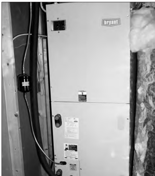
a two-stage gas furnace. Both of these furnace designs vary the heat output of the gas burners depend-
