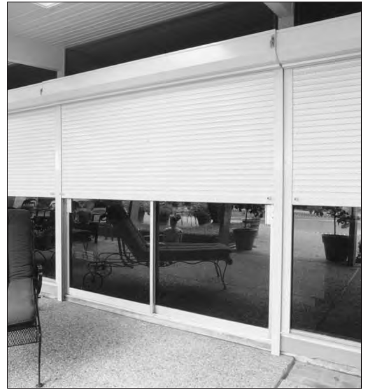
These rolling shutters are partially opened over sliding glass doors.
