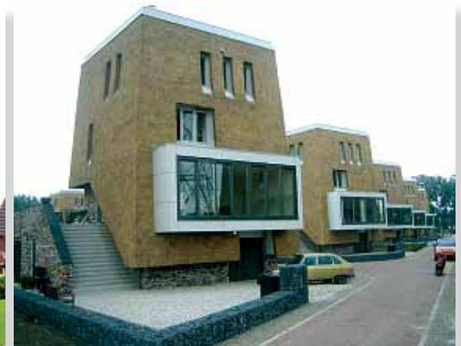
These buildings exemplify the modern style of reed construction. Reed can also be fitted to exterior walls, as in these examples from the Netherlands. Photo: The Dutch Federation of Thatchers.
