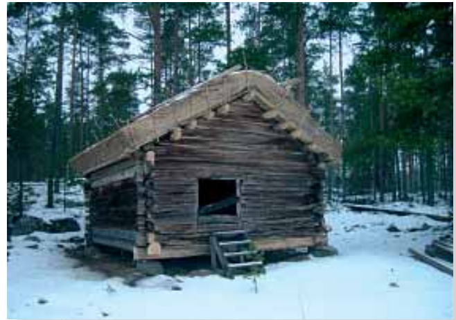
Restored reed roof of a barn. Rymättylä, Southwest Finland. Photo: Markku Hyvönen.
