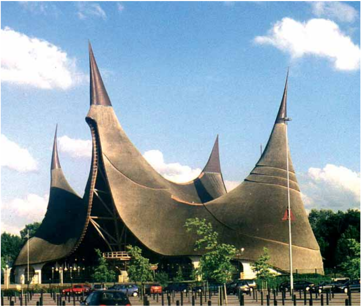
Obviously the world's largest single reed roof is located in the De Eferling amusement park. This roof measures over 5,000 square meters. Photo: The Dutch Federation of Thatchers.
