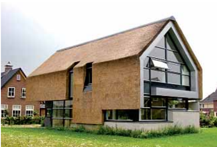
These buildings exemplify the modern style of reed construction. Reed can also be fitted to exterior walls, as in these examples from the Netherlands. Photo: The Dutch Federation of Thatchers.
