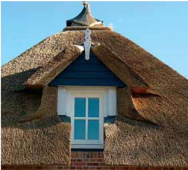
Beautiful detail on a mitre box. Photo: The Dutch Federation of Thatchers.
