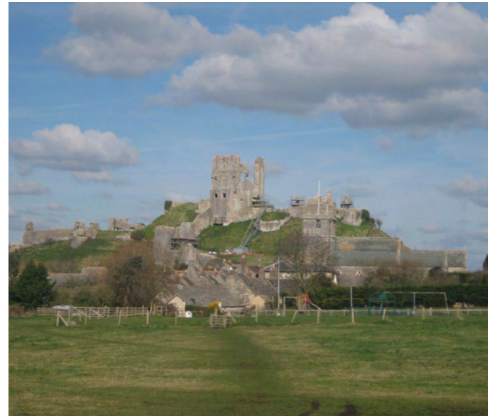
1. The Castle is a Grade 1 listed building
