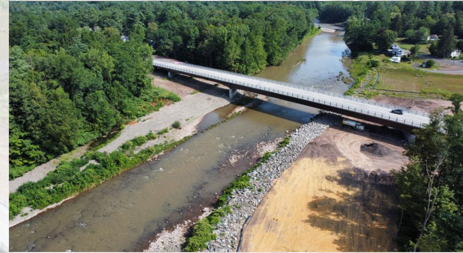
Drone view of new bridge over the Esopus Creek. Note the wide span which allows for wildlife movement and reduces the potential for flooding.
