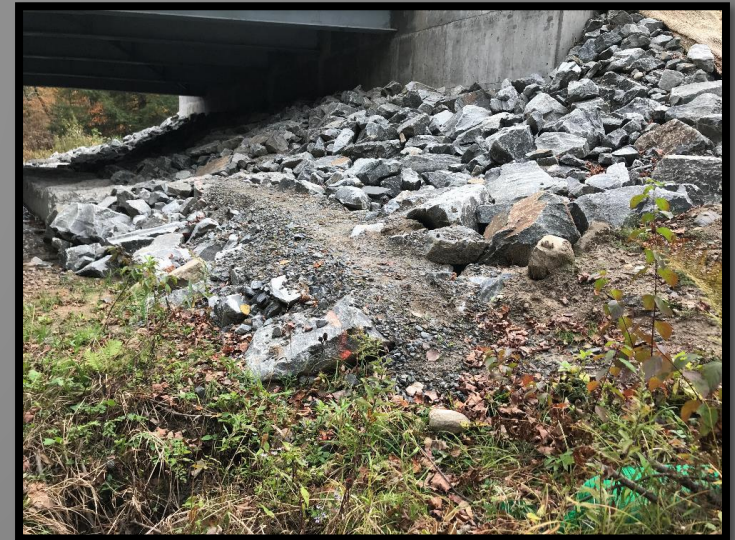
North end of the completed terrestrial critter trail on native soils.
