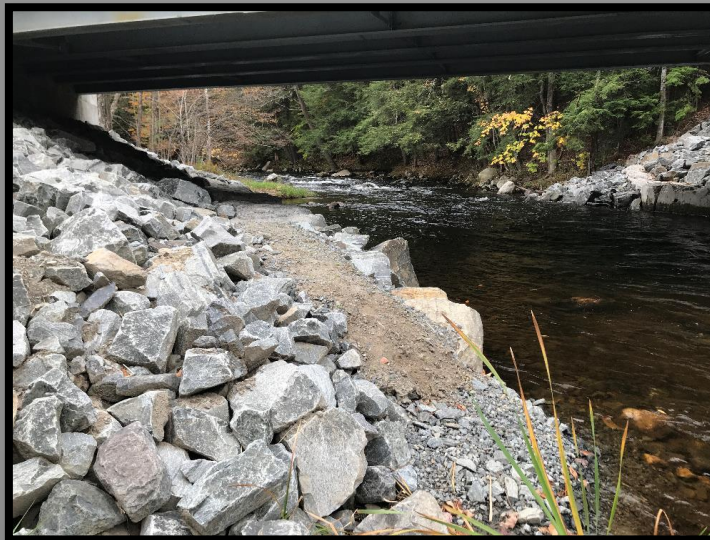
View north along the constructed terrestrial critter trail under Rte 10A.
