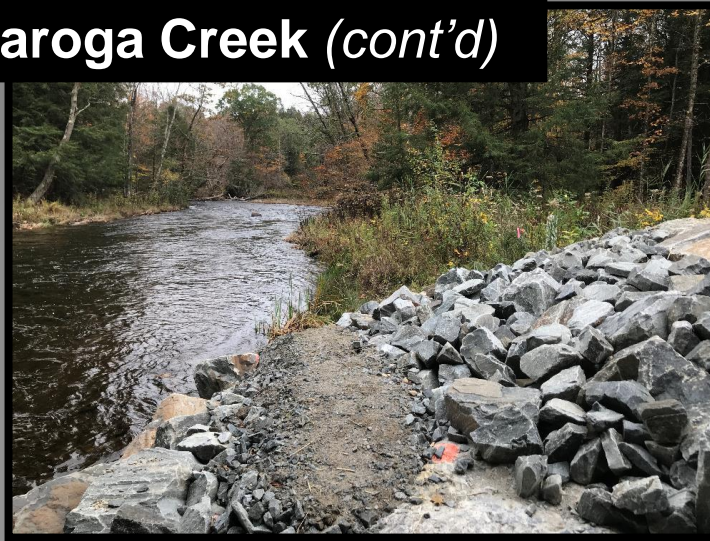
South end of the constructed critter trail adjacent to the Caroga Creek bank.
