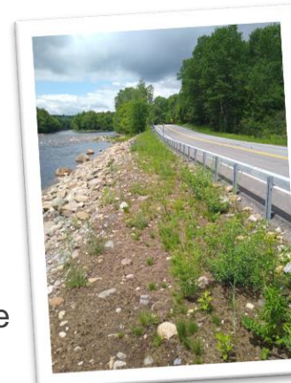
Looking south at ProGanics site in Summer 2021. Site has only about 50% ground cover.
