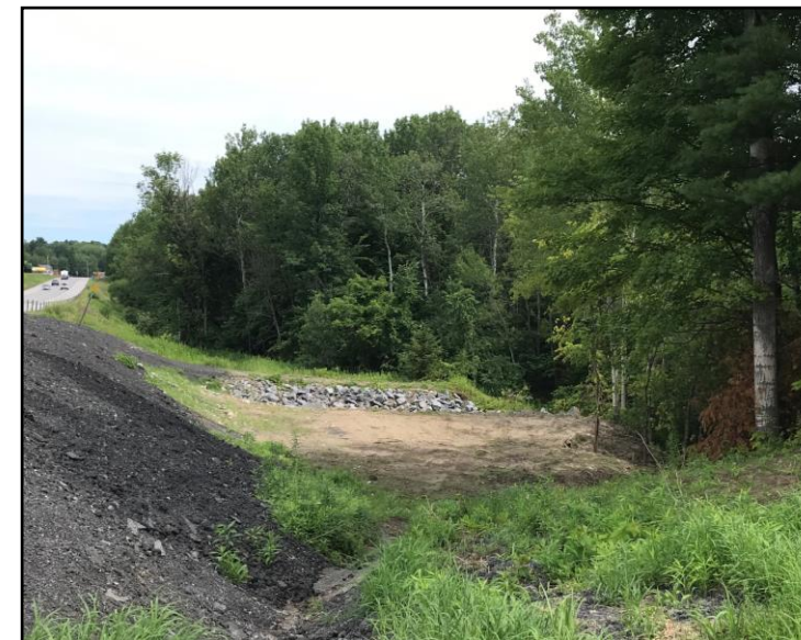
Image of reconstructed slope before turf establishment
