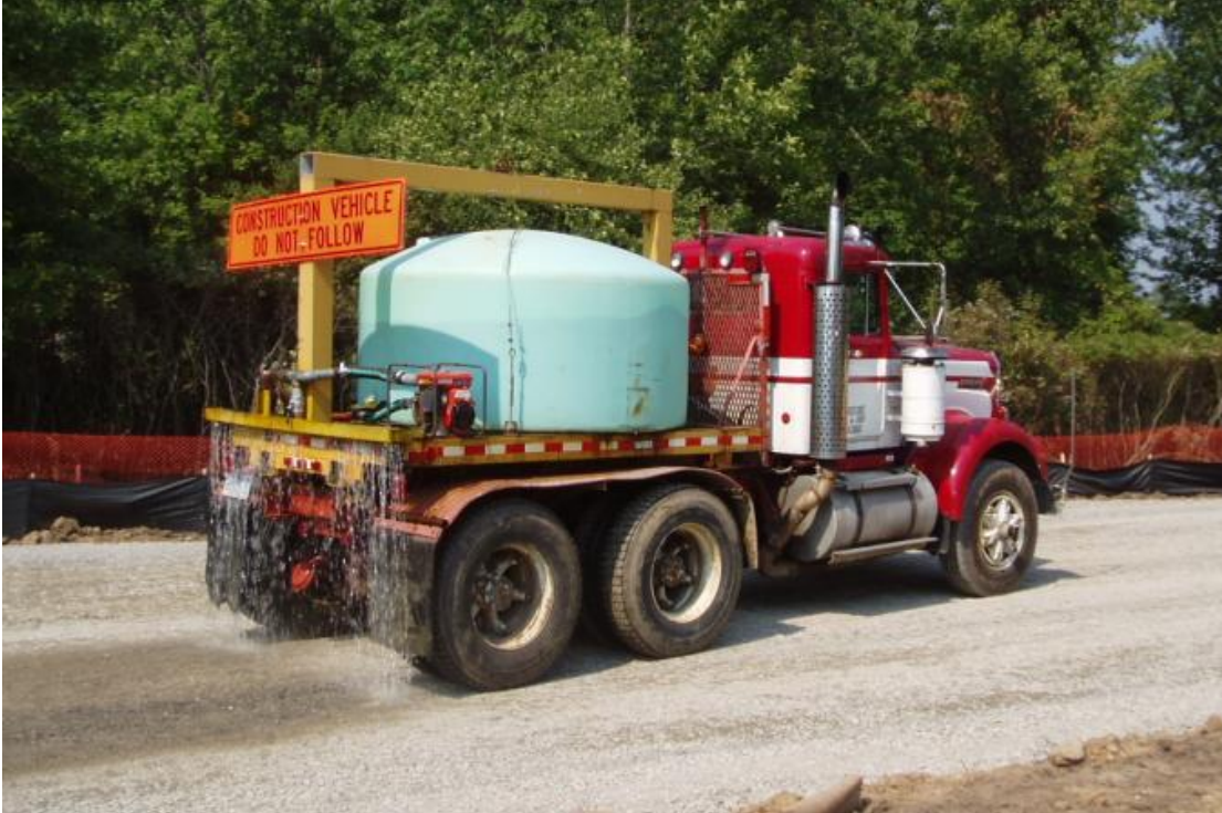
Figure 28 Water Being Applied By Water Truck
