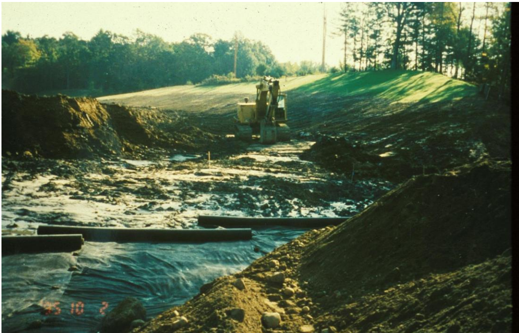
Figure 21 Construction Lift Backfilling Undercut of Embankment Foundation Utilizing a Geotextile Separator
