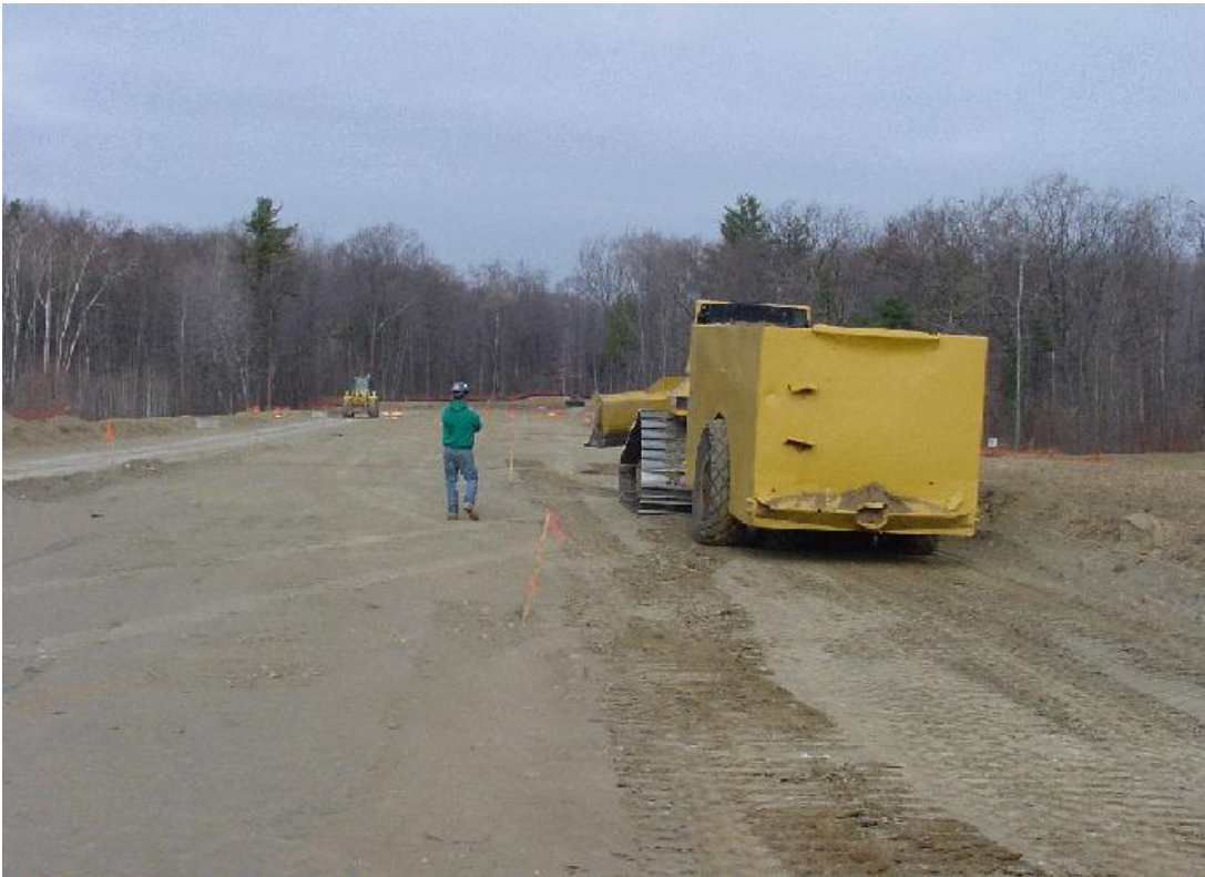
Figure 29 Normal, Stable Embankment Construction
