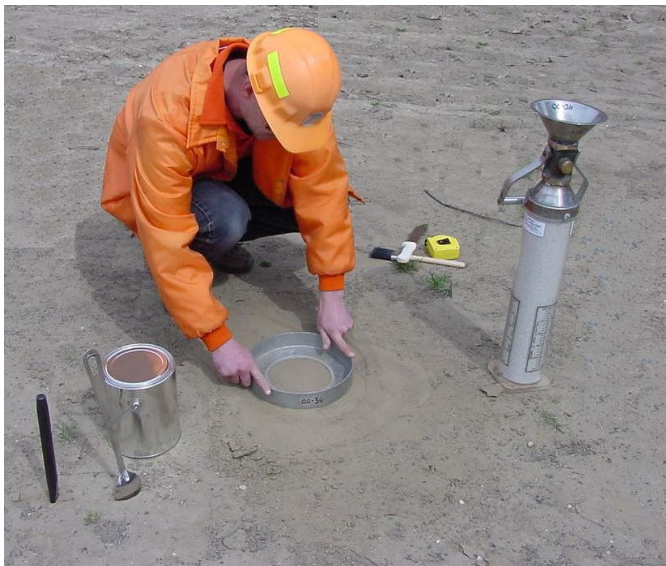
Figure 25 Compaction Control – Volumeter
