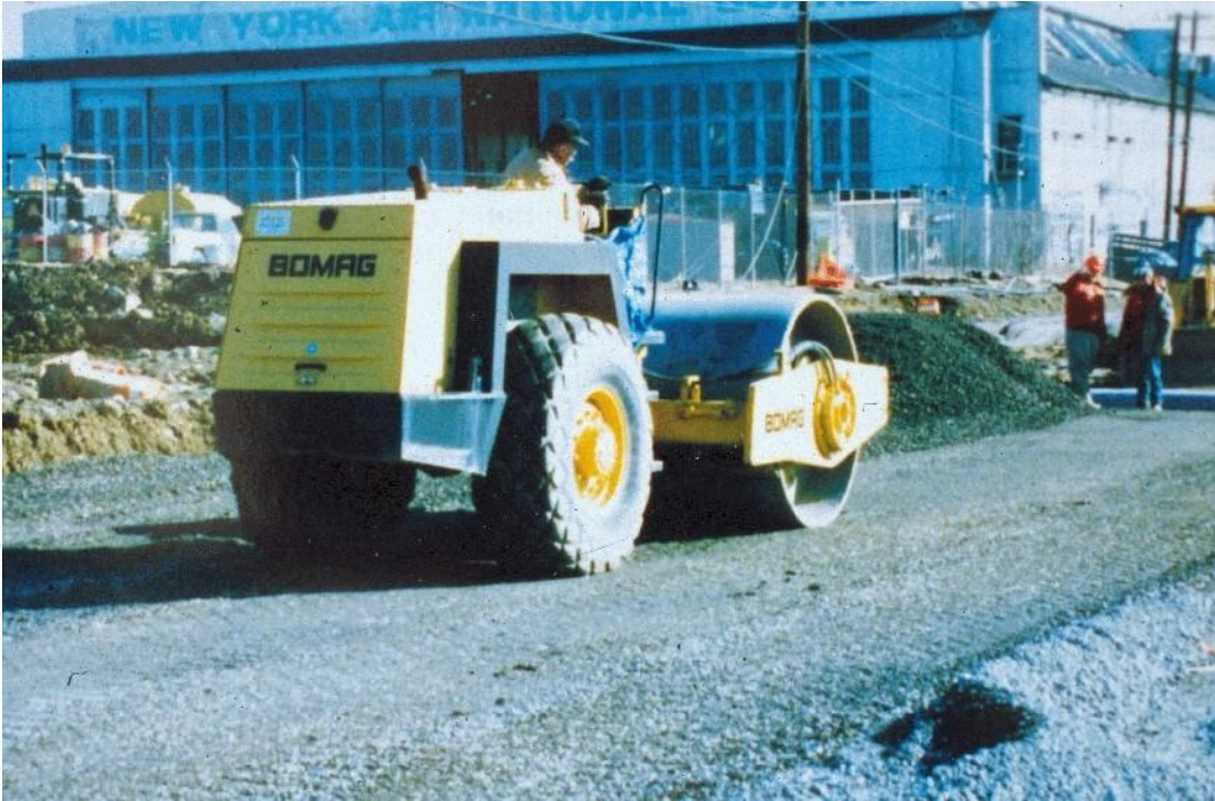
Figure 24 Normal Compaction Operation – Vibratory Drum Compactor
