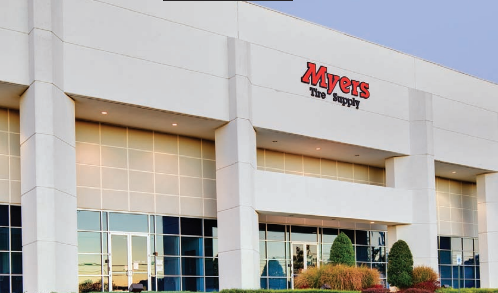
Memphis Distribution Center
