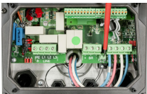
Fig. 27: Connecting the motor cables
