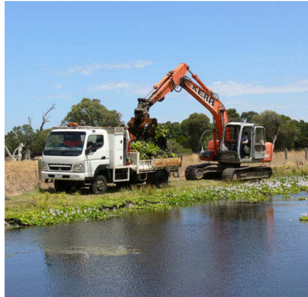
Excavator loading plant material directly onto truck
