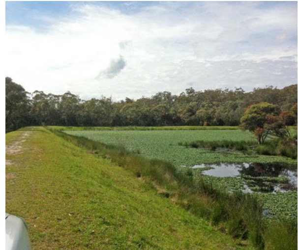
Water hyacinth invading the water treatment plant at Wyong South
