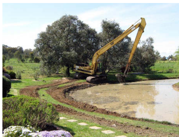
Excavator scooping out mud and sediment to remove the seed bank
