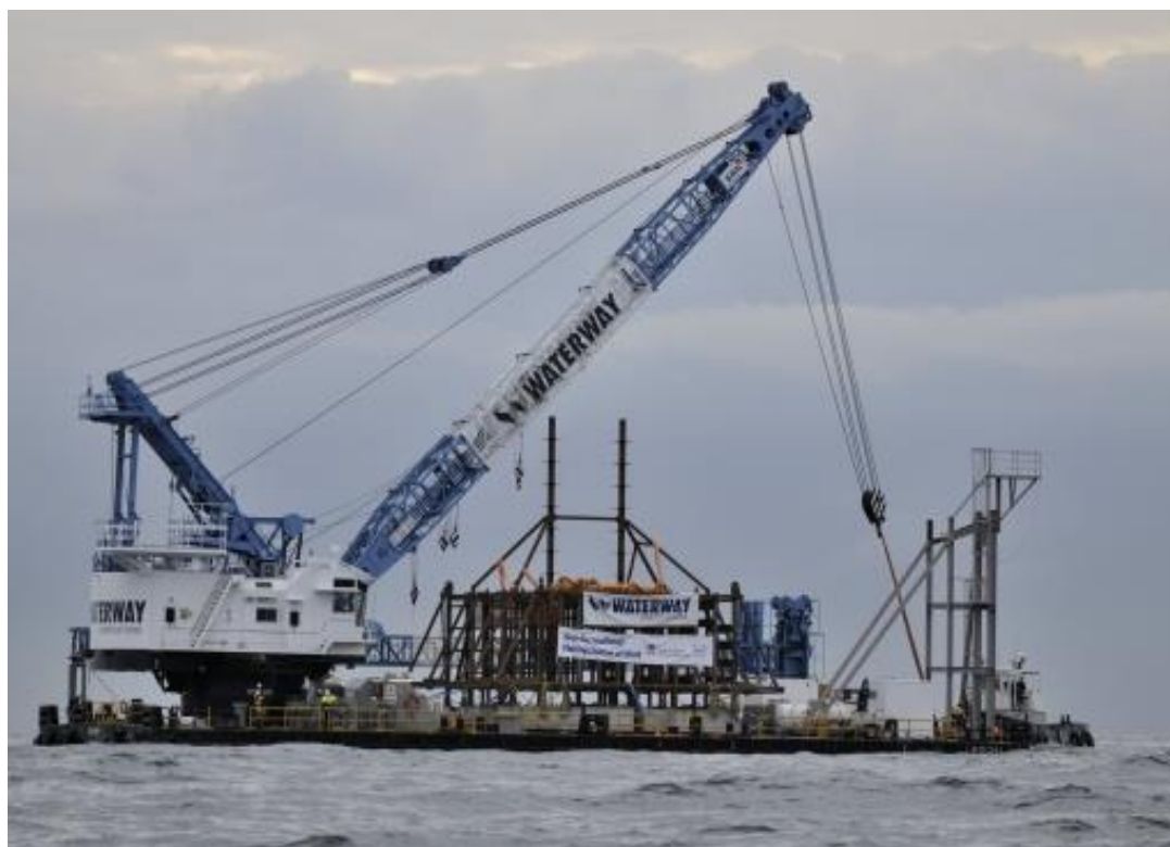
Figure 2 Deploying the offshore artificial reef
