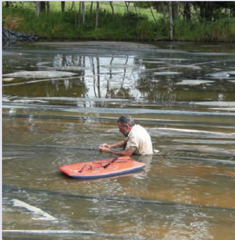
Plastic zip ties were used to join the roped edges back together.
