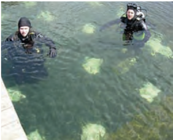
Blanket secured to bottom with sandbags
