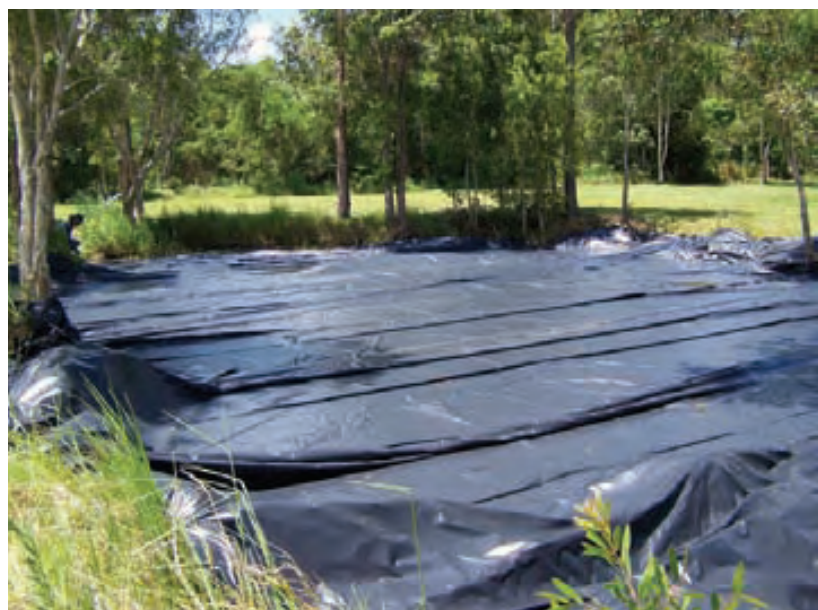
A floating blanket constructed from builders' black plastic
