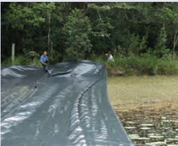
Sheets were overlapped to create a complete light barrier.
