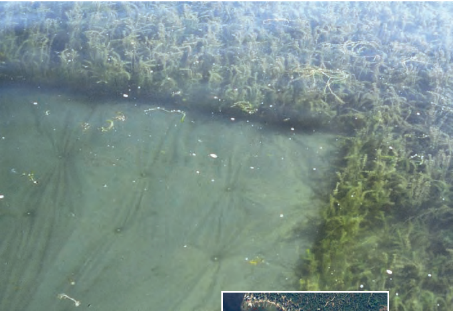
A section of benthic blanket installed over water milfoil
