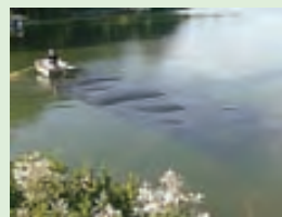
Installing a Lake Bottom Blanket® © Lake Bottom Blanket
