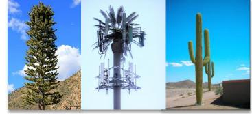
Fig. 1, Concealed Cell Tower Examples – The images above show a few examples of how cellular tower sites can be concealed to reduce impact on sensitive visual or cultural landscapes.
