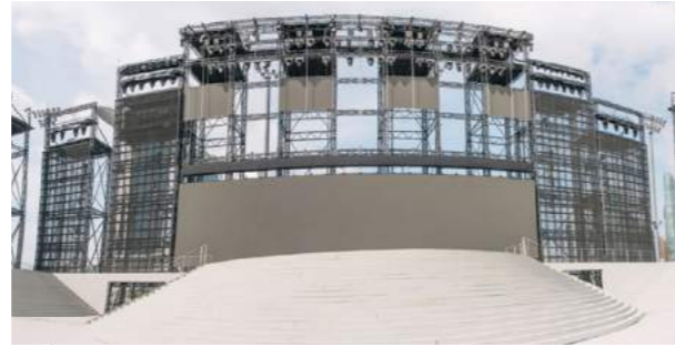
The two-tier stage of NDP 2014 was the largest ever to be constructed in NDP's history, with a capacity of 1,800 performers and their props, 18 towers and 10 elevating platforms.
