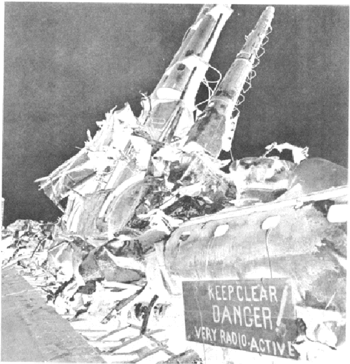
Figure 26. Damaged USS Skate (SS-305) on 3 July following Test ABLE.
