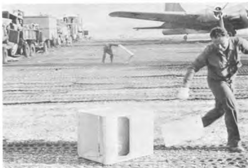
Figure 22. Second filter holder comes free from top filter. Man in background tilts top filter unit from another drone. Junk revetment is at right, SANDSTONE.
