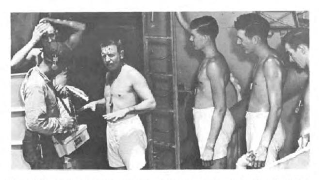
Figure 24. Decontamination monitor locating and marking spots of radioactivity on personnel returning from a radex area, REDWING.
