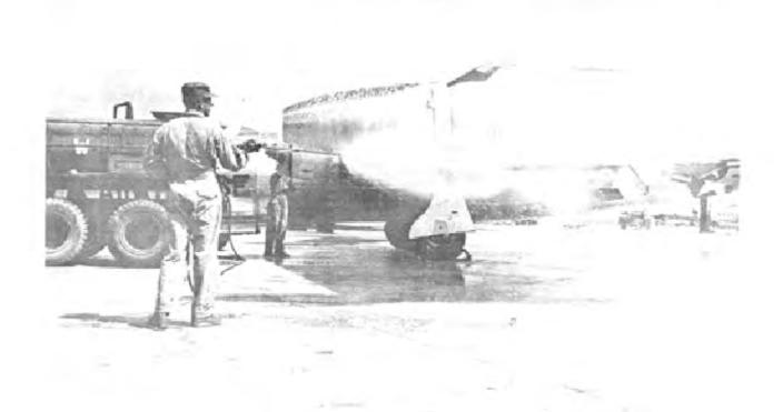
Figure 32. Decontaminating a B-57 sampler aircraft after flight through a nuclear cloud, REDWING.
