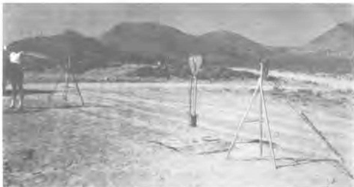
Figure 5-8. OVERALL VIEW OF MONITORING RIG.
