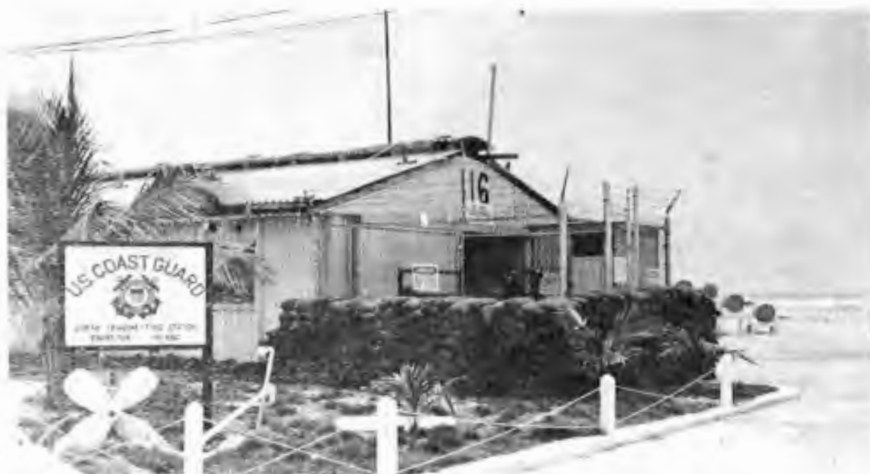
Figure 56. Transformer at U.S. Coast Guard Loran station on Enewetak Island sandbagged in preparation for HARDTACK, OAK.
