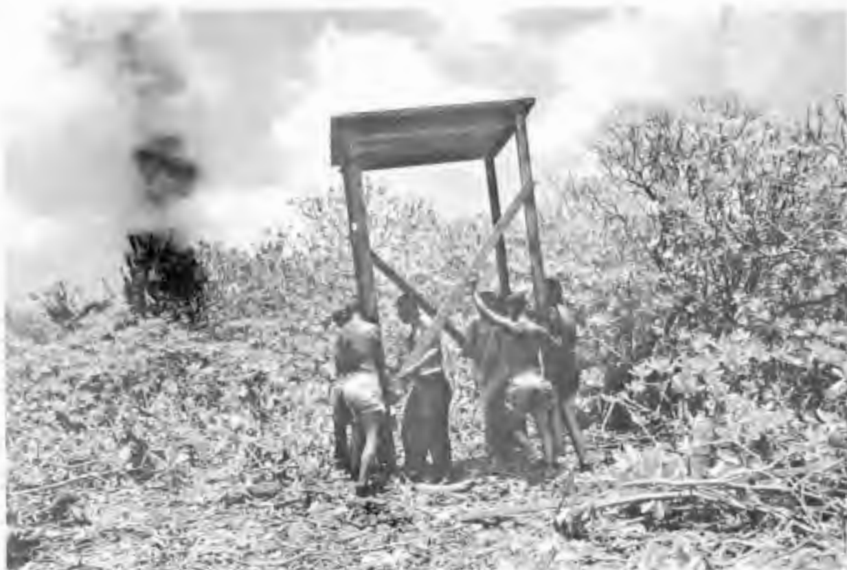
Figure 8. Small photo tower being built on Mut Island, Enewetak Atoll, in heavily vegetated area, 1958.
