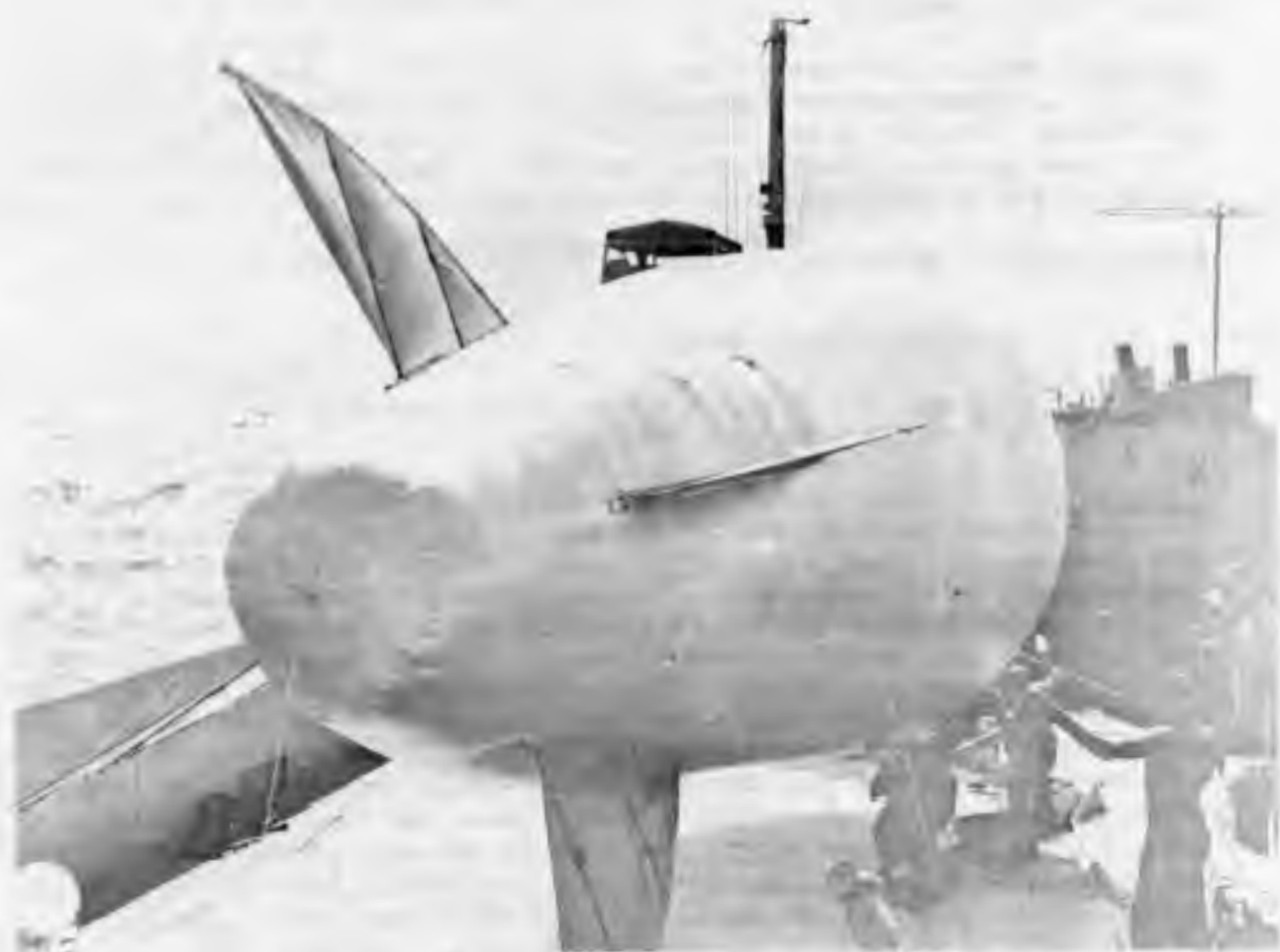
Figure 29. Project 1.2 balloon in LCU inflated for raising, HARDTACK.
