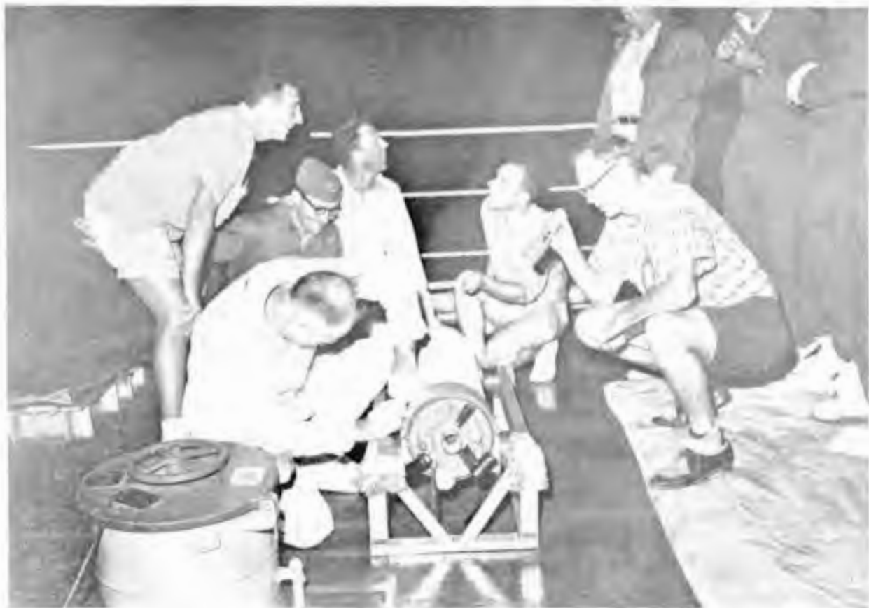
Figure 26. Protective clothing worn by USS Lansing (DER-388) crewmembers (standing) after recovering a radioactive pod that had been exposed to the high-altitude HARDTACK, TEAK shot. Project 8.6 personnel are examining the pod.
