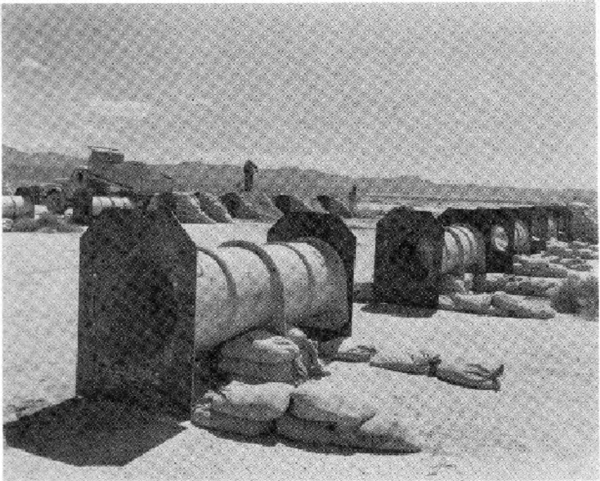
Figure 4-2: RAT CYLINDERS USED IN PROJECT 4.2 AT SHOT ENCORE
