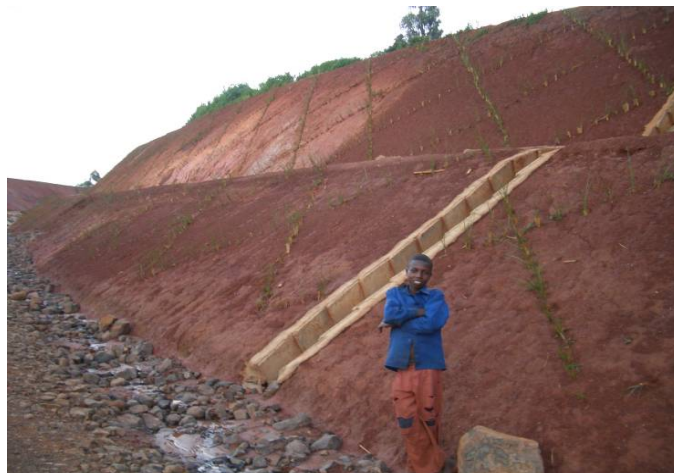
Figure 1.1 Non-native grasses are being used to prevent the roadsides from eroding under heavy rains. Photo: A.B.S. 29 Sept. 2005 from road between Nekemte and Assosa.
