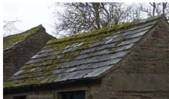
Slate and sandstone roofs
