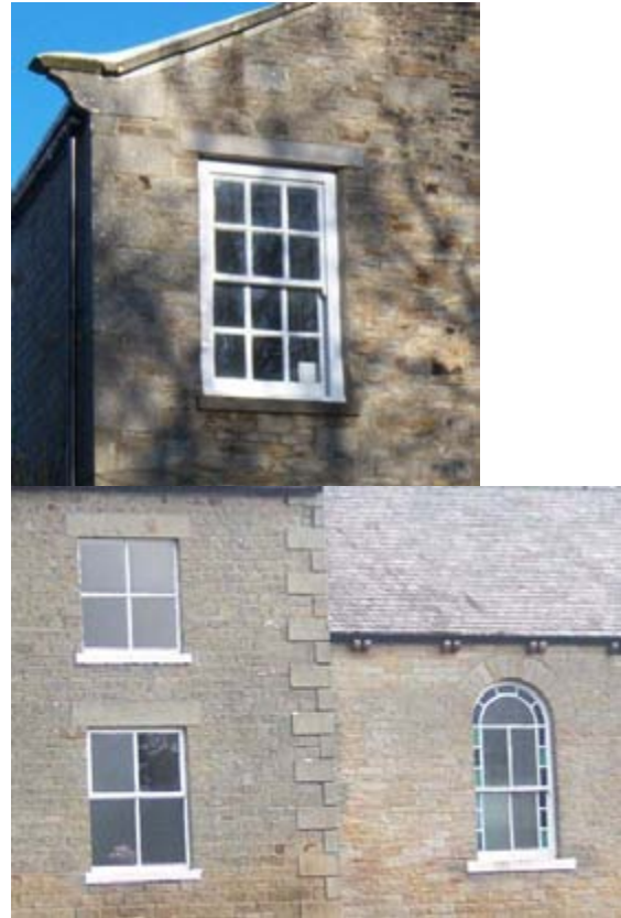
Traditional windows in original, historic openings.
