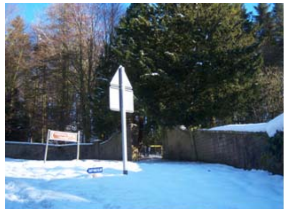
Walls and gate piers opposite Low Lodge.
