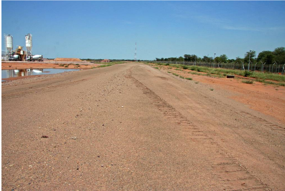
Figure 5: View to the west indicating the disturbed area south of the road where it is recommended the pipe should be laid.
