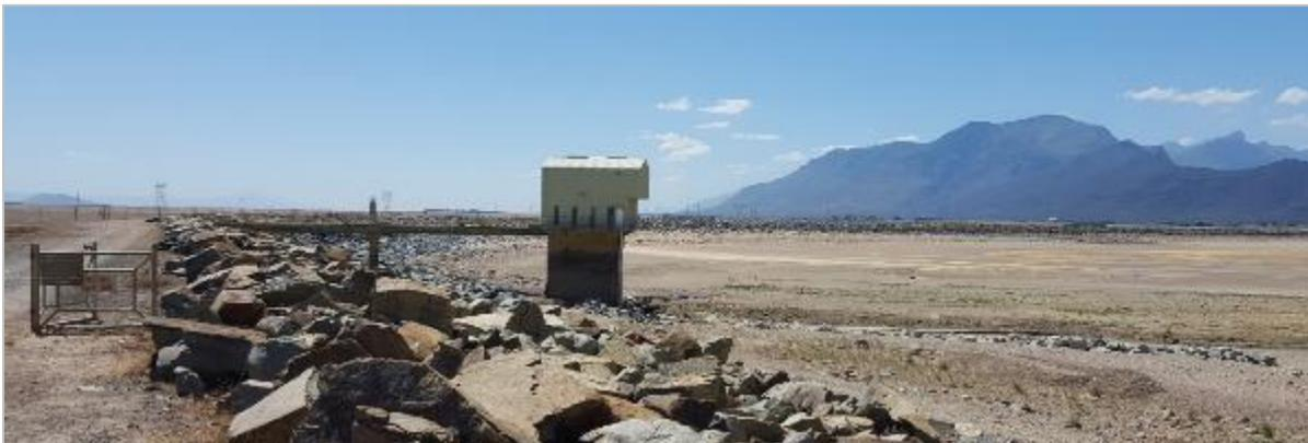
*Figure 55: One of the intake towers located on the Dam*
