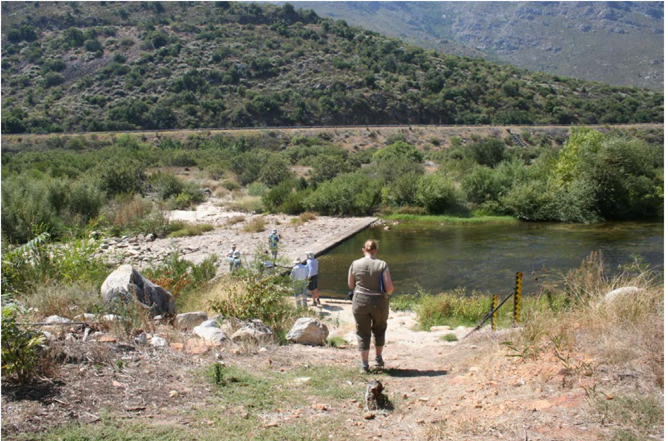
Figure 12. Present weir and off-take from Breede River at the downstream entrance to Mitchell's Pass.
