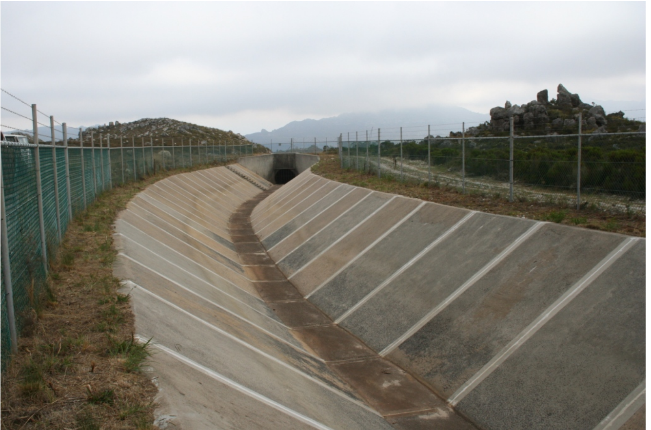
Figure 5. The existing canal and pipeline from the Rockview Dam illustrated here is designed to take all the anticipated additional flows resulting from either of the proposed Campanula Dam schemes thus no further disturbance is anticipated along this section.
