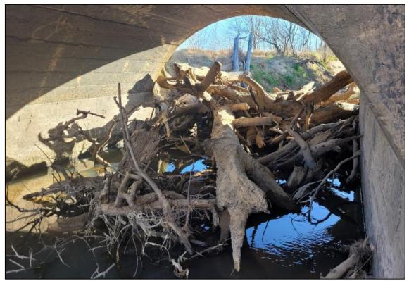
Figure 3-84 Debris below a large road culvert across the incised portion of the floodplain.
