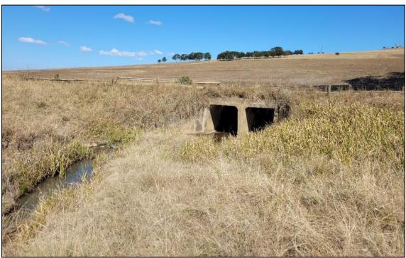
Figure 3-126 View of the road culvert associated with the R61 which has led to the formation of a small headcut erosional feature upstream of the culvert. The headcut has not progressed too far due to the shallow bedrock layer within the system
