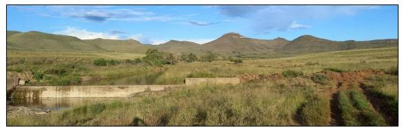
Figure 3-138 An erosion-control concrete weir in a small valley bottom in the Loodsberg foothills, likely constructed several decades ago through Department of Agriculture's soil conservation initiative.
