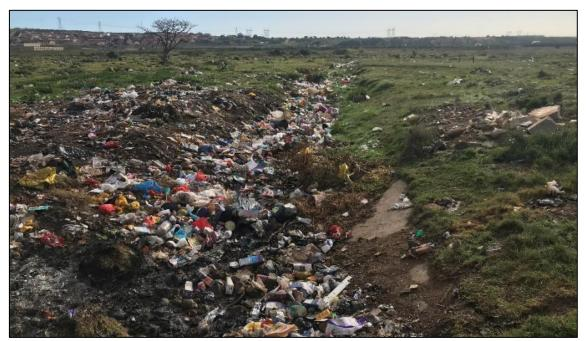
Figure 3-36 One of the many stormwater canals that conveys stormflows into the Chatty River Wetlands. Many of these canals have been totally blocked by the litter and debris, causing them to overtop into inhabited areas, potentially posing a health risk to those living nearby. In addition, the canalised stormwater conduits that are not blocked were observed to, in some cases, have resulted in erosion and scour of the downstream wetland.
