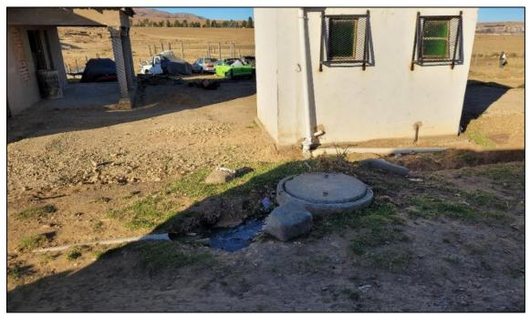
Figure 3-92 Surcharging manhole with the sewage being directed towards the wetland
