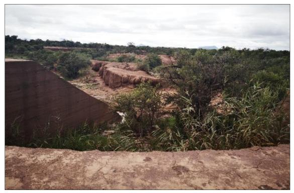
Figure 3-50 View of the erosion gully downstream of a weir
