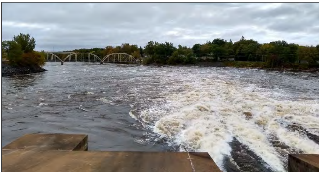
Figure 4.9.1-2: View Downstream of the Sartell Dam
