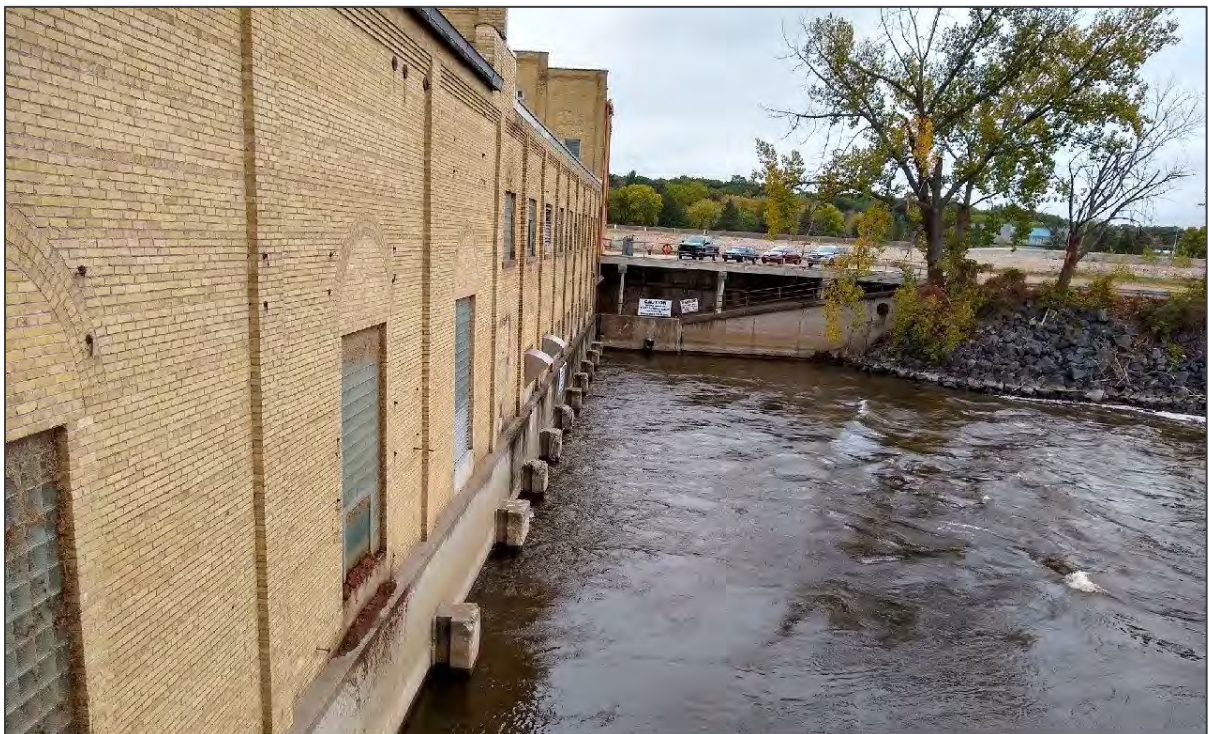
Figure 4.9.1-4: Sartell Project Powerhouse and Tailwater
