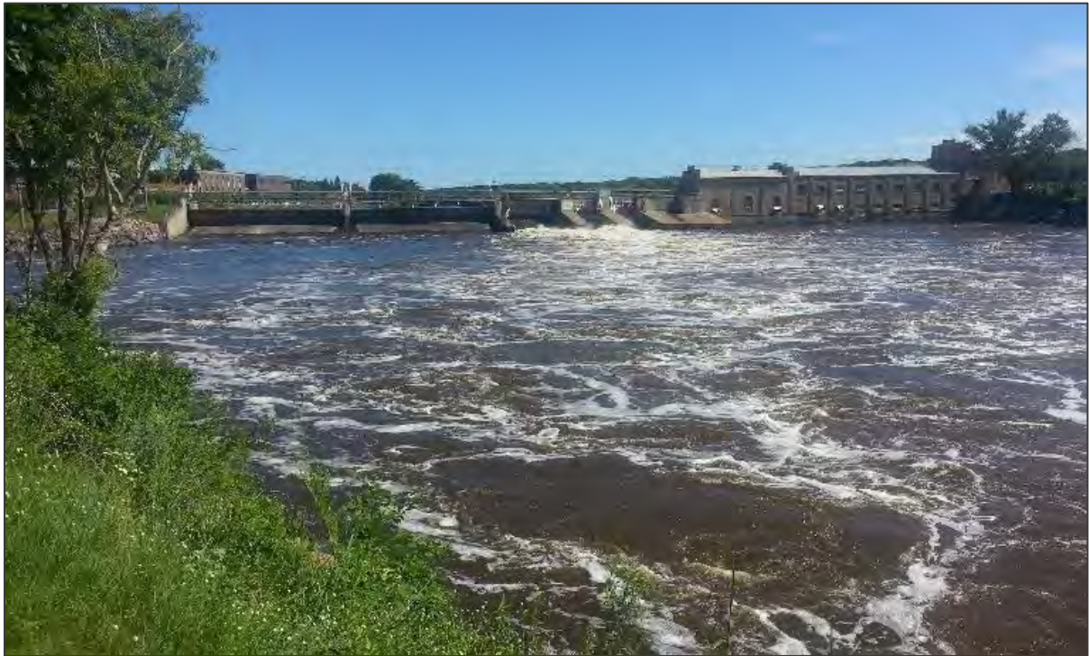
Figure 4.9.1-3: View of the Sartell Dam from Veterans Park
