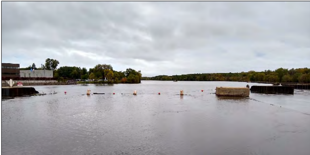
Figure 4.9.1-1: View of the Project Reservoir Upstream from the Sartell Dam
