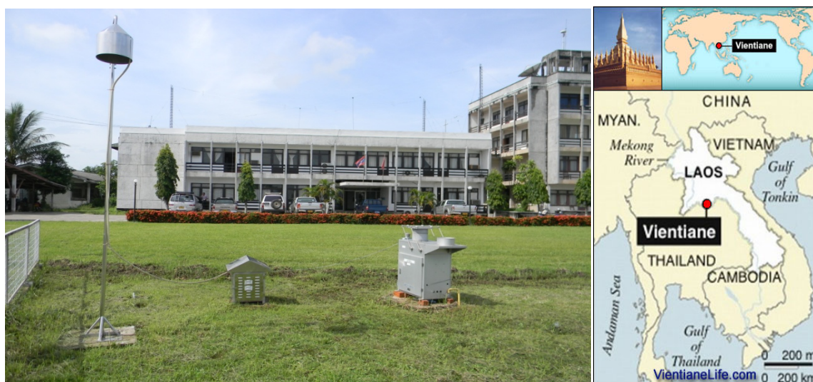
Figure 5.1.1. Monitoring station for wet and dry deposition.
