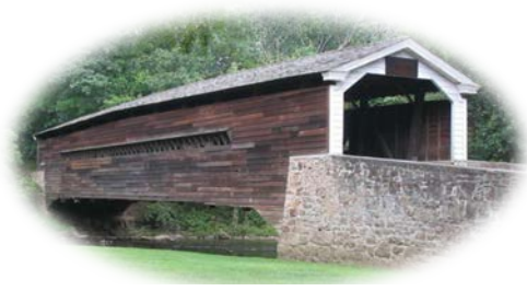
Rapps Dam Covered Bridge
