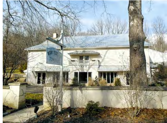
West Pikeland Township building. Web source image
