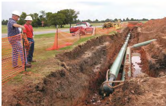
Pipeline under construction. Image credit: U.S. Air Force
