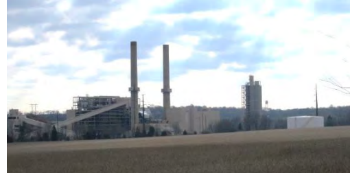
Cromby Electric Generating Plant in East Pikeland Township
