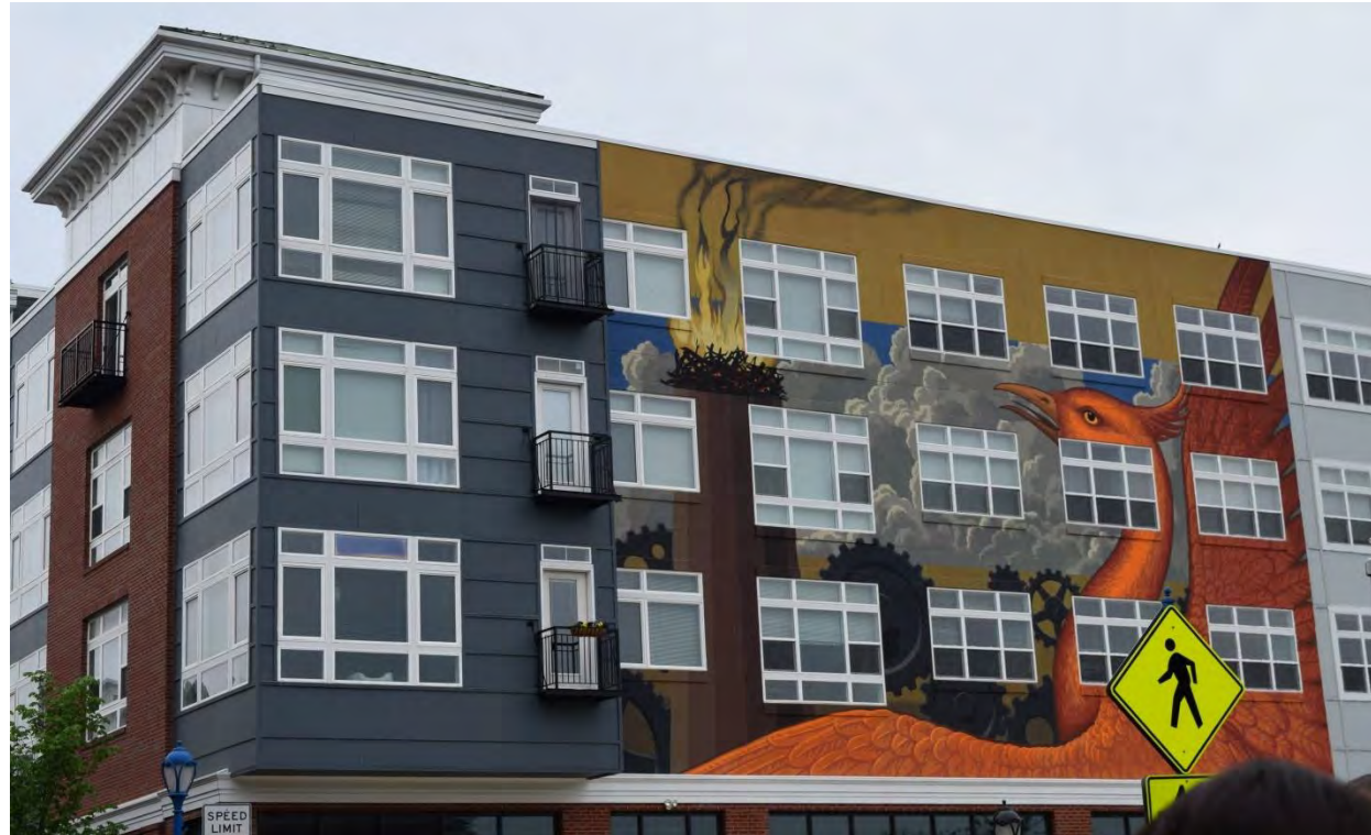
New apartment building in Phoenixville. The Borough's relatively dense built environment supports more apartment developments. Image credit: Borough of Phoenixville
