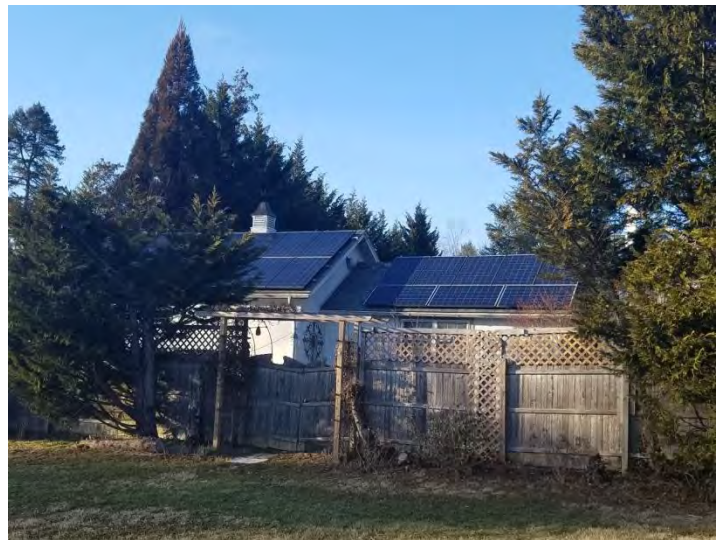
Solar PV Panels on a Residence
