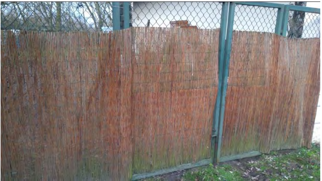
Fence covered with reed, copyright Zoo Lodz
