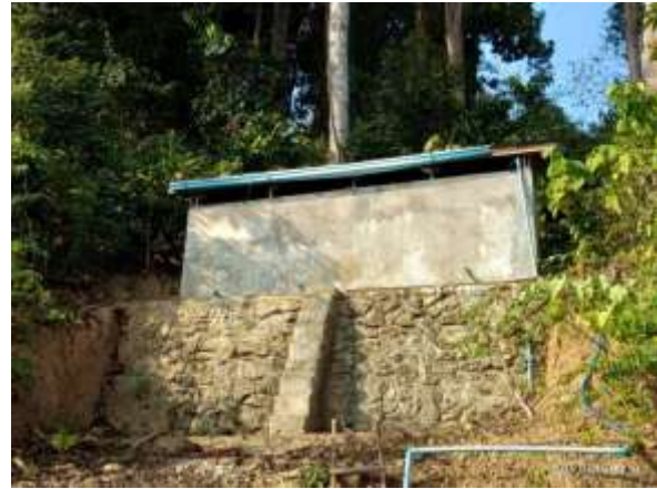
Figure 5-36 Water Storage Tank
