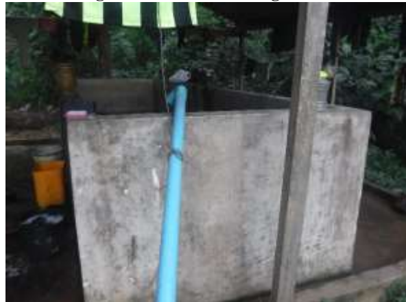
Figure 5-38 Water Storage Tank
