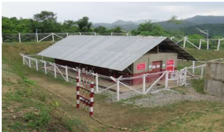
Figure – 14: 50 Tons Magazine (outside the factory compound)
