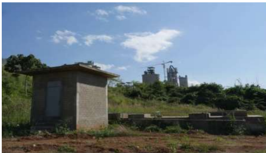
Figure – 106: Sewage treatment
