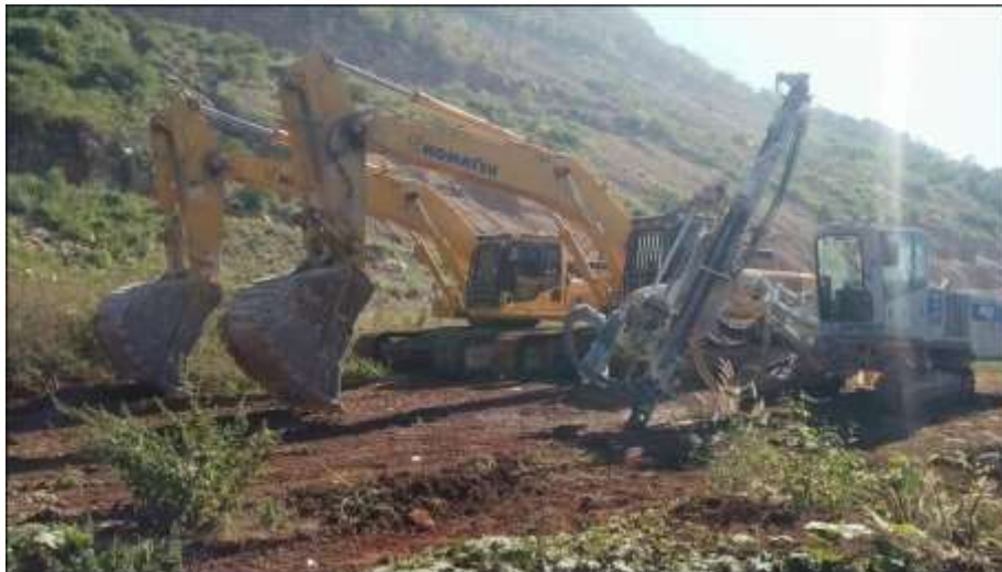
Figure – 38: Heavy machinery
