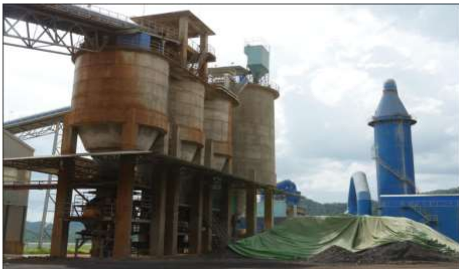
Figure – 26: Conveyor and four raw material bins (alumina and silica clay, Laterite and limestone) raw meal silo is background
