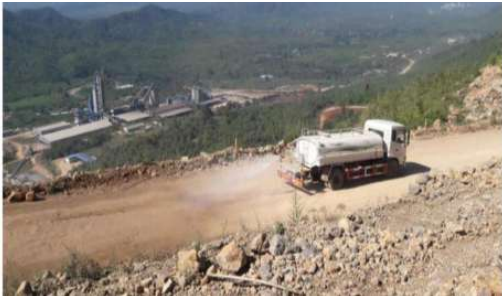
Figure – 99: Spraying water for suppression of dust at the site (one of the options), especially along the dusty haulage road
