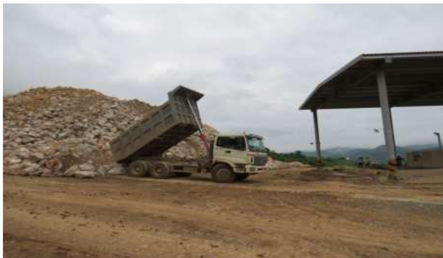
Figure – 102: Stockpiling of limestone
