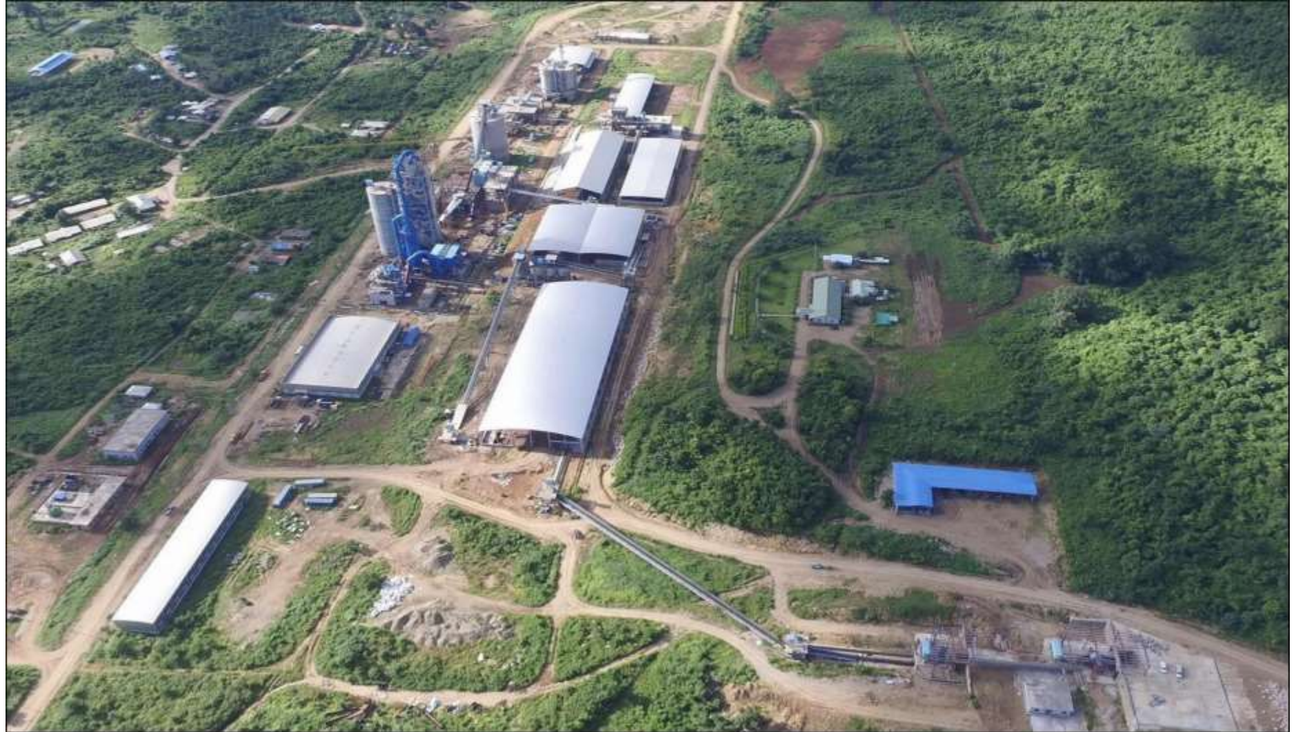
Figure – 7: Overview of project site (factory and premise)
