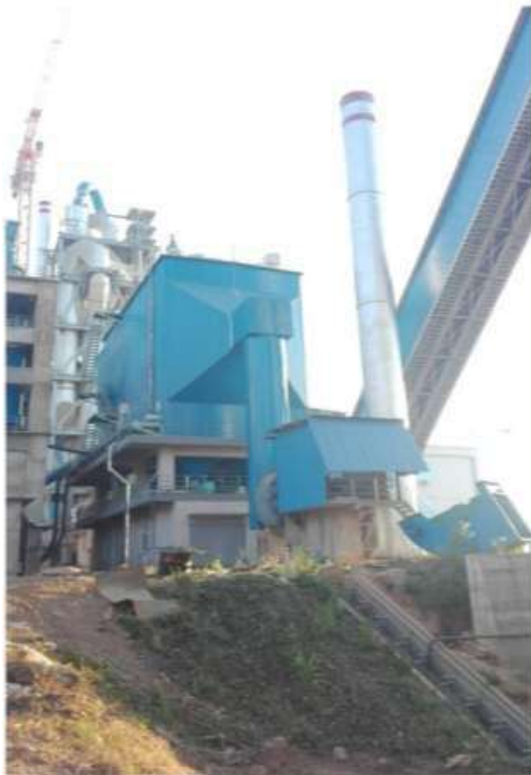
Figure – 48: ESP unit
