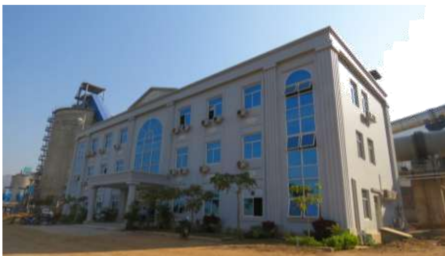
Figure – 41: Building with CCR room, the laboratory and clinic
