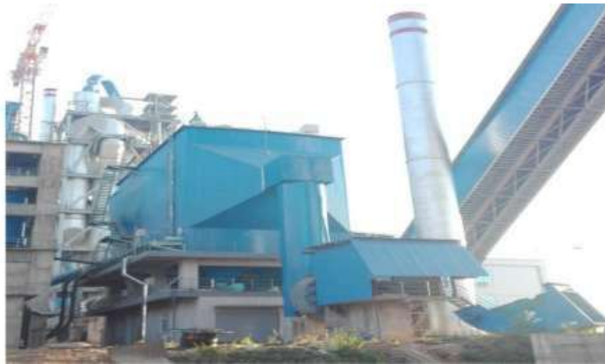
Figure – 101: ESP unit
