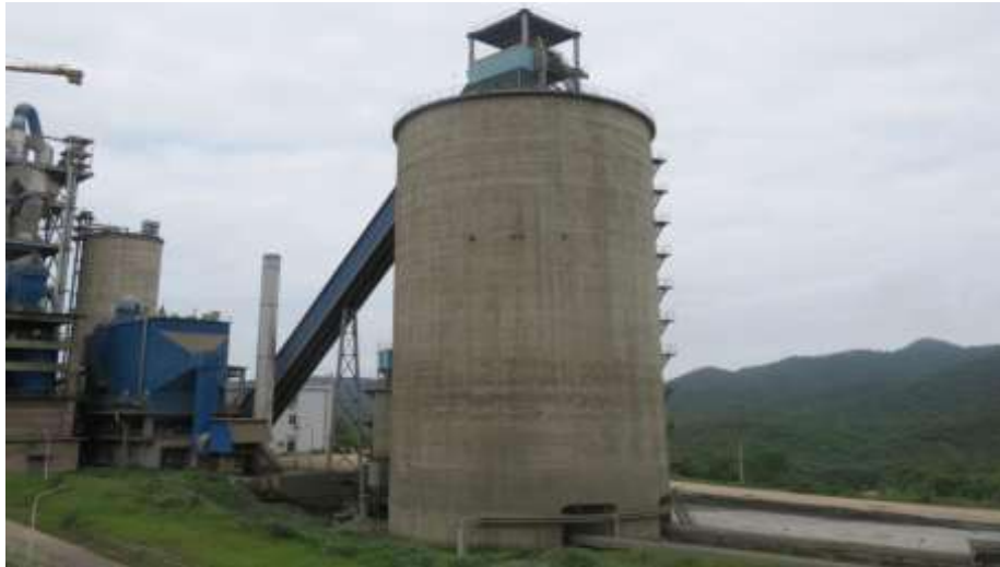
Figure – 30: Clinker silo
