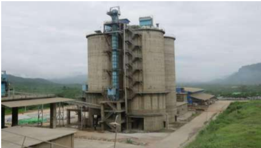
Figure – 31: Cement silo
