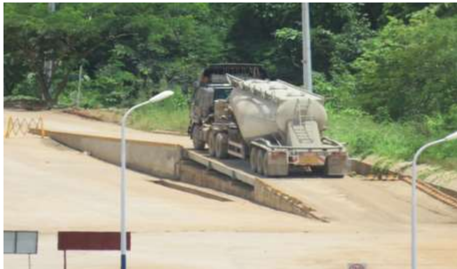
Figure – 13: Weighing bridge (with a cement mixer in it, outside the factory compound)
