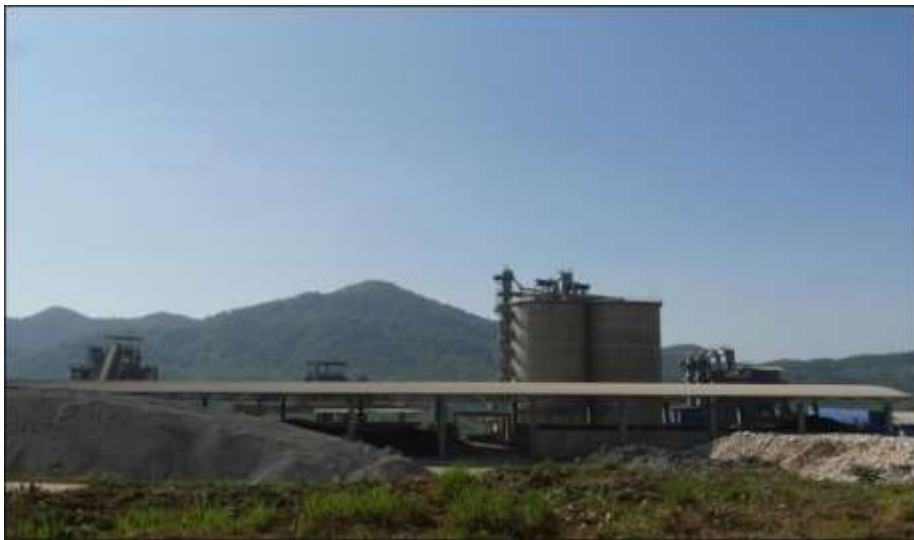
Figure – 22: Gypsum and Additive Crusher and Storage Shed
