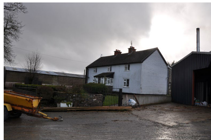
View of the east-facing front façade of the property showing windows on both storeys.
