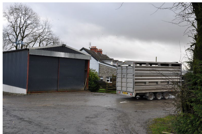
View of the north-facing gable-end of the building, and dormer windows on the western 'rear' façade.
