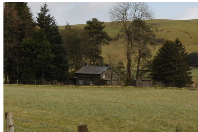
View to the north-western and south-western façades of the property, showing the conifer woodland to the north-west.
