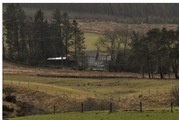
The north-north-east facing façade of the property with windows on both storeys.
