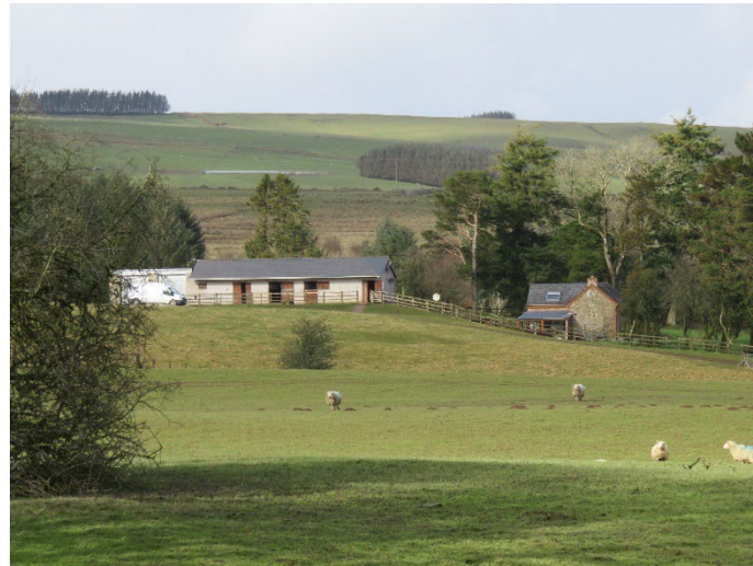
View from the south-east, showing the stable outbuilding situated on more elevated ground to the west of the property.
