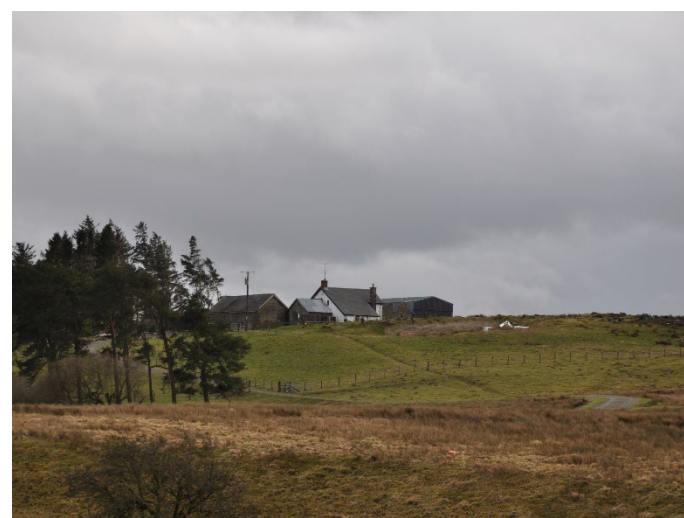
View to the north-eastern and north-western façades of the property from near Custogion Brook
