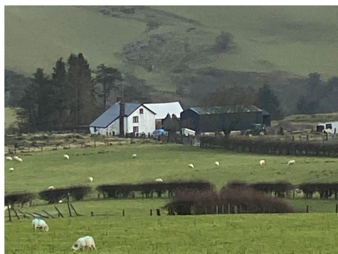
View to the north-west and south-west façades of the property from a track to the west (within the Site)
