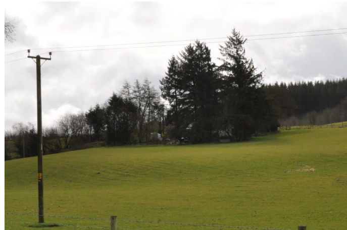
The north-east facing gable end of the property, visually enclosed by dense hedgerow boundaries of mature conifer trees.
