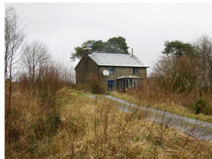
View towards the south-east facing front of the property.
