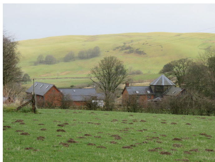
View of the north-western façade of the property, taken from the minor road through David's Well.
