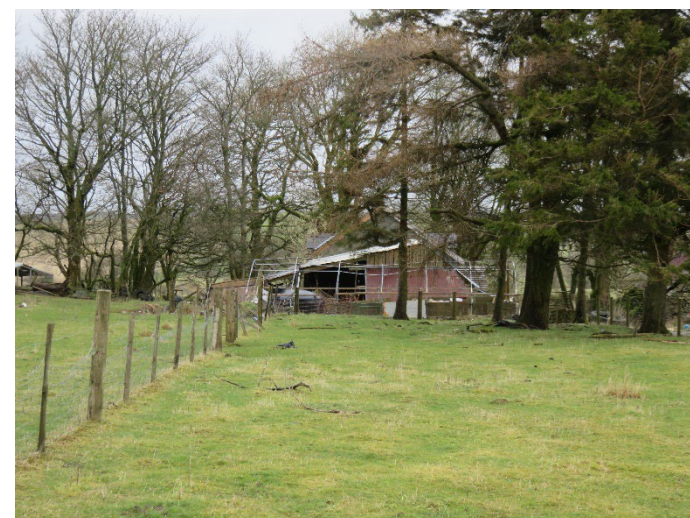
View showing the southern gable end of Ffordd Las.
