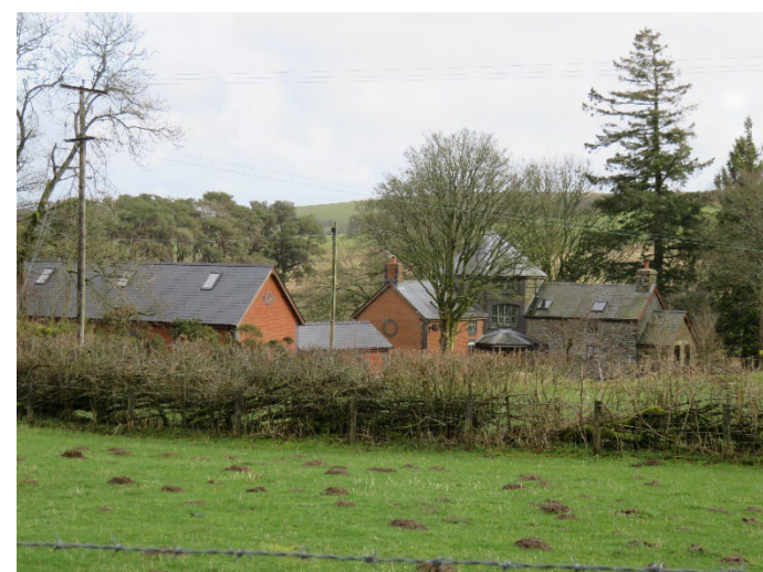
View of the north-western façade of the property.
