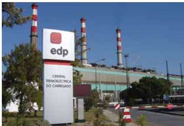
Thermolectric Power Station
