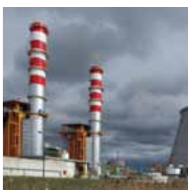
Ribatejo Thermoelectric Power Station
