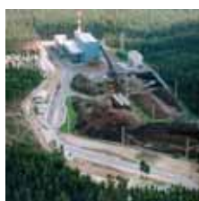
Mortágua Forest Waste Power Station
