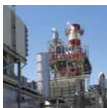
Energin Cogeneration Power Station
