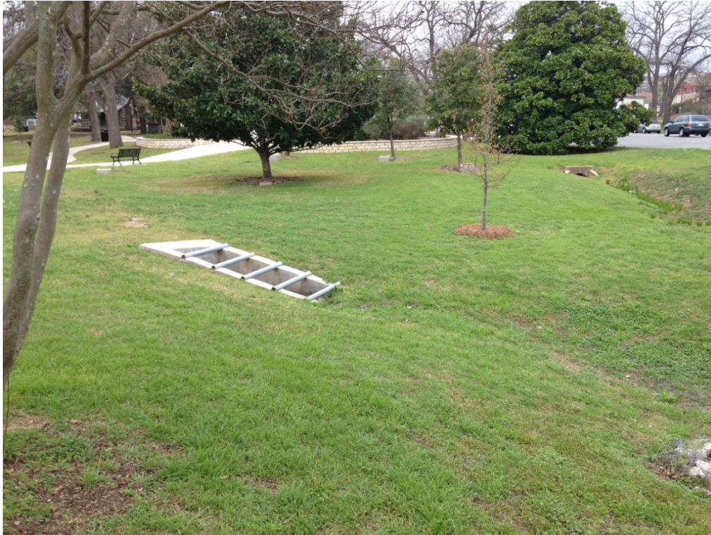
Figure 3-1 Two Storm Sewer Outfalls and Proximity to Veramendi Park Amenities
