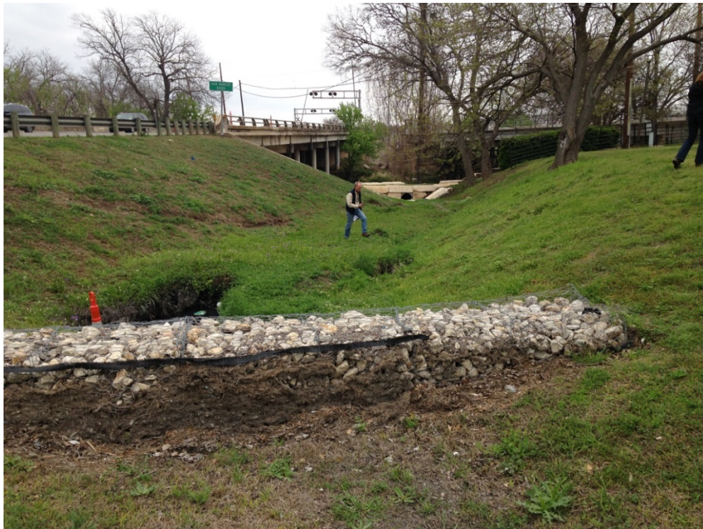
Figure 3-2 Gabion Grade Control Structure, Trail, Steep Slopes, Trees, Hopkins Street Bridge
