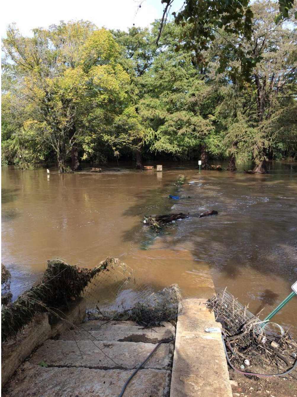
Figure 11 Cypress Island bridge on October 31st, 2015.
