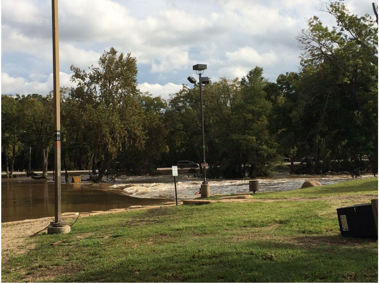
Figure 12 Rio Vista Dam on October 31st, 2015.
