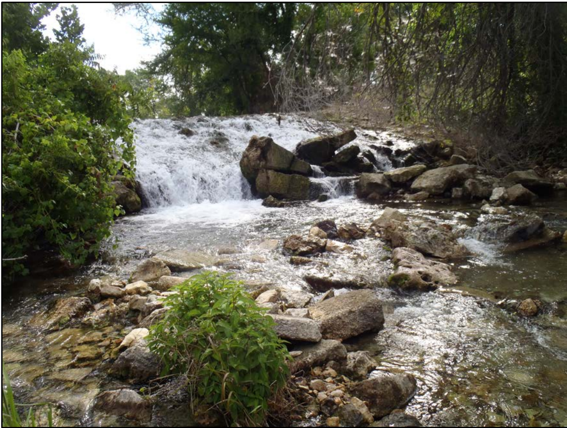
Figure 9: Spring Lake Dam Spillway on July 27, 2022.
