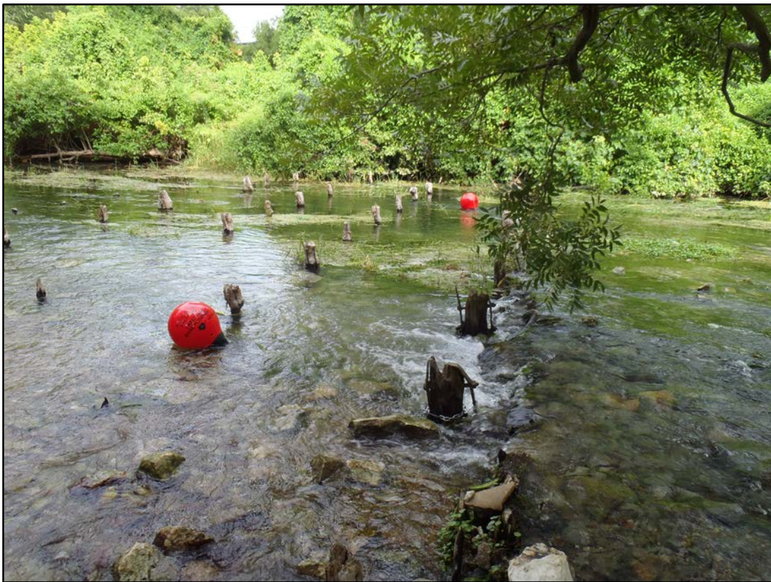
Figure 10: Spring Lake Dam water level on July 27, 2022.
