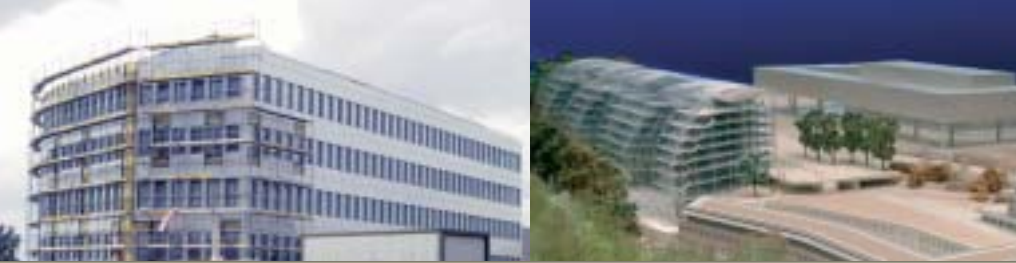
New Building at Hamm
