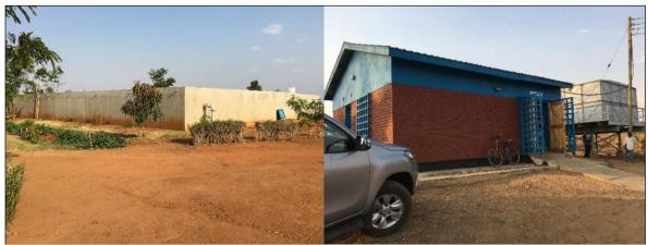
**Figure 1.2:** Existing Sosola reservoir (Left) and pump house and collector tank (right) for the Balaka water supply system
