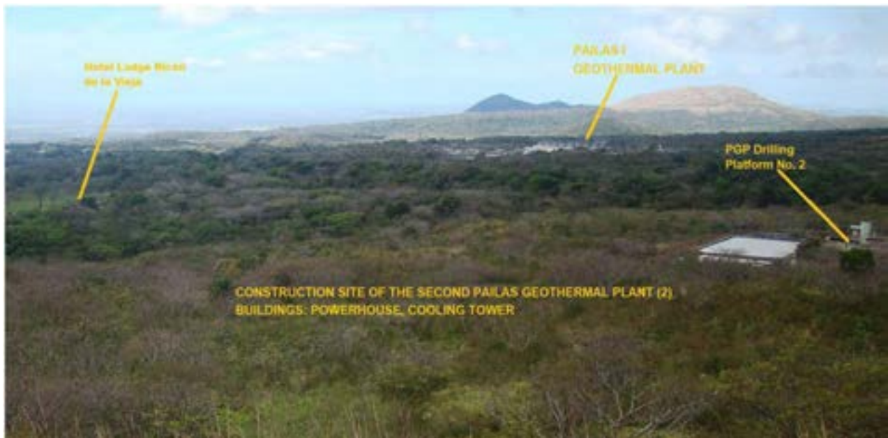
Photograph 5. 2 Panoramic view of the construction site of the additional geothermal plant
