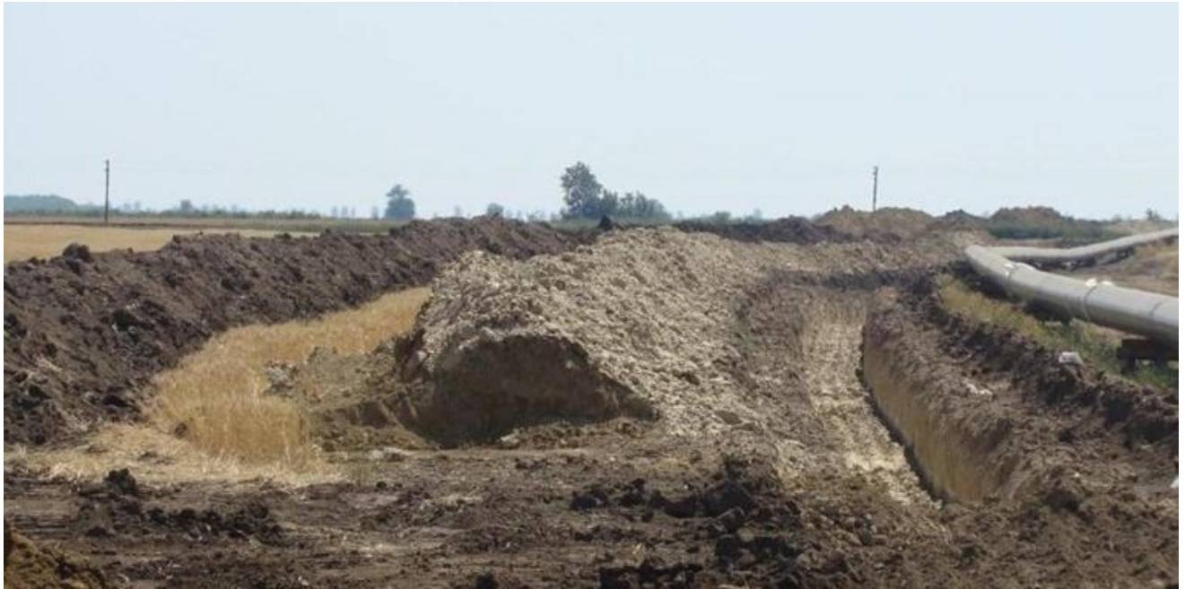
Figure 4.3 Image of a working strip for gas pipeline laying
