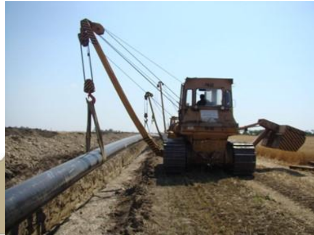
Figure 4.5 View from construction site
