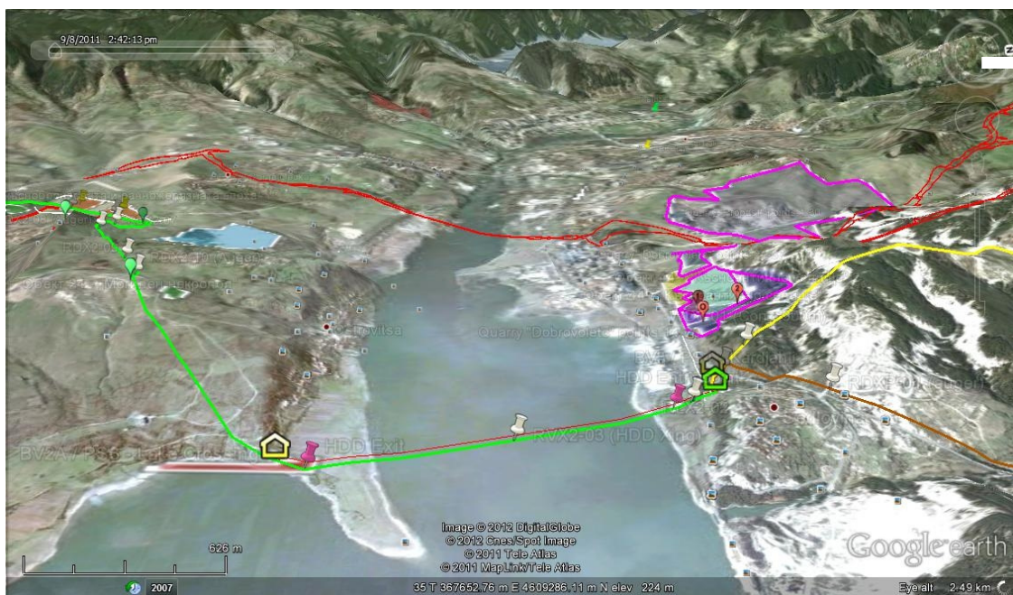
Fig. 1.2.1.2-1 – Crossing of Studen Kladenets Reservoir at Kardzhali (of length 1 500 m) indicated by the green line across the reservoir
