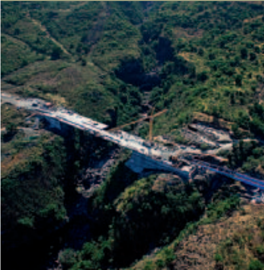
The Grande Ravine viaduct on Reunion Island.
