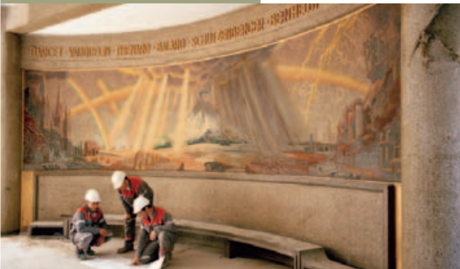
Renovating the Collège de France.
