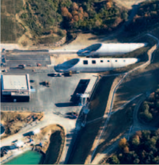
Dummy tunnel mouths at the exit of the Perpignan-Figueras high-speed line.
