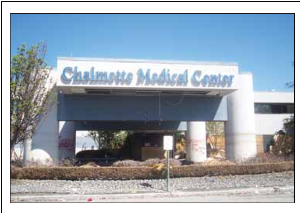
Figure 2-5. Damage at Chalmette Center
