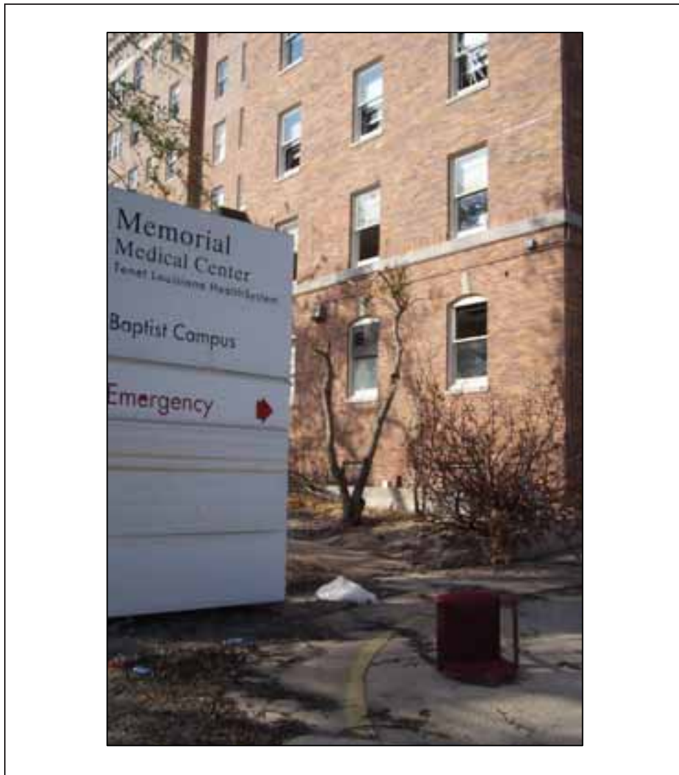
Figure 2-3. Damage at Memorial Medical Center
