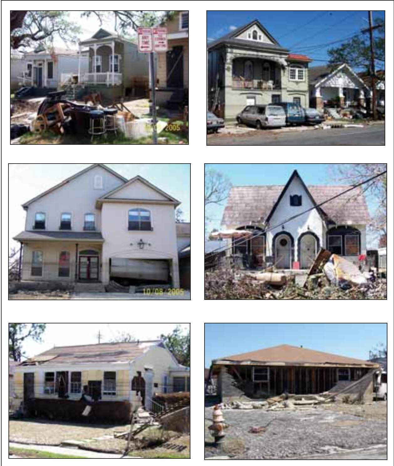
Figure 5-3. Housing in Orleans and St. Bernard Parish was Substantially Damaged by Flooding
