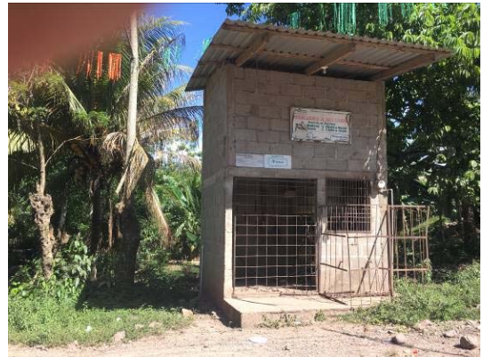
Former water potabilization system in the community of Juncal
