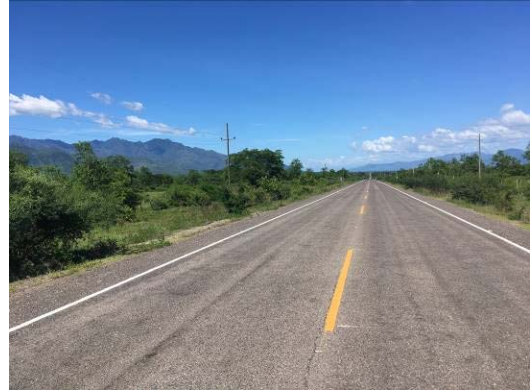
Asphalted road, fence, telephone cables and electrical line
