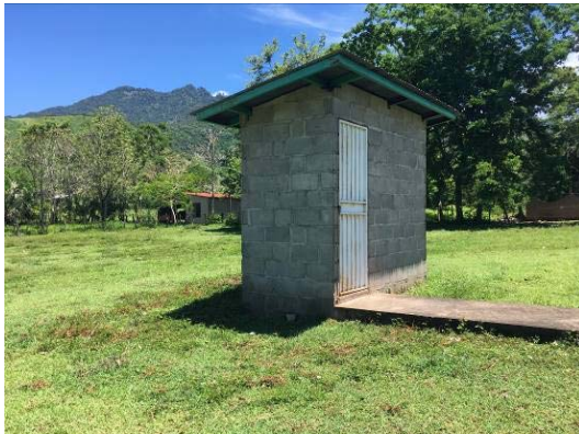
CREL Salinas Gonzales y Asociados: WC with septic tank system by filtration to the subsoil
