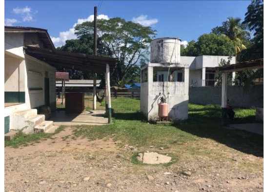
Aerial water storage tank in CREL Eberto Chirinos Ponce
