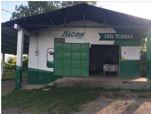
Main building of CREL Tejeras
