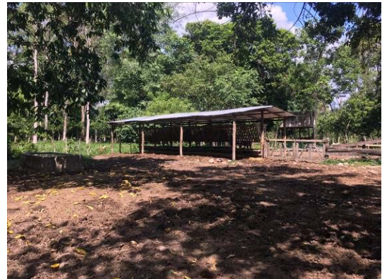
Cowshed under construction in farm #108
