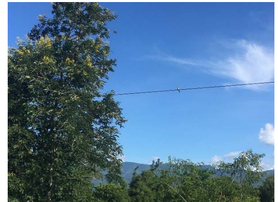
Bird in electrical line
