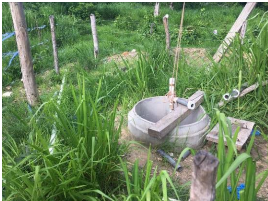
Groundwater well in farm #71 providing water cattle consumption
