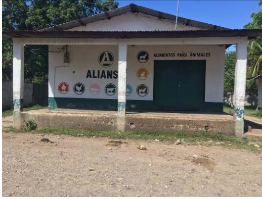
Main building of CREL Eberto Chirinos Ponce
