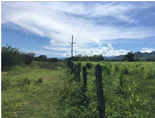
Electrical line and fence next to the road
