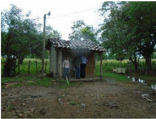
Protection stall for underground well in Leopoldo Duran Dueñas.
