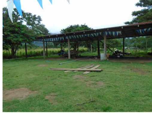
Rancho Don Juan, using underground water source.
