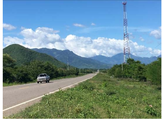
Road and communication antenna
