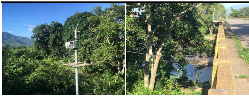
Figure 5.10 View of the vandalized meteorological station in the Aguan River
