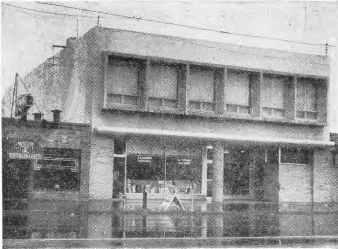
The State Crime Commission calls this building a $200,000 "fortress." At 313 San Pablo Avenue, El Cerrito, it is the office and home of William M. Pechart.—Tribune photo.
